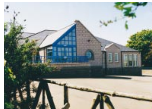
Improved capital asset - Letham School extension
