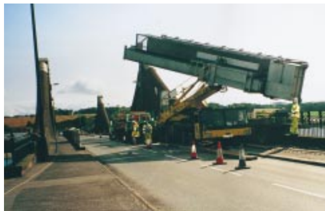
Mobile bridge inspection access platform at South Esk Bridge, Montrose
