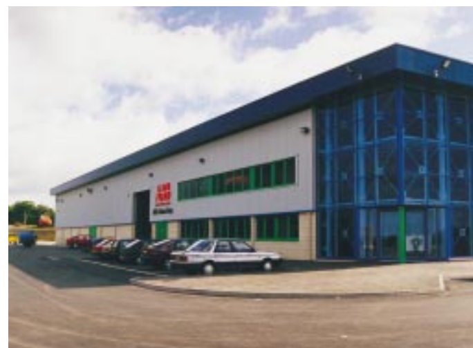
Factory development at Brent Avenue, Montrose
