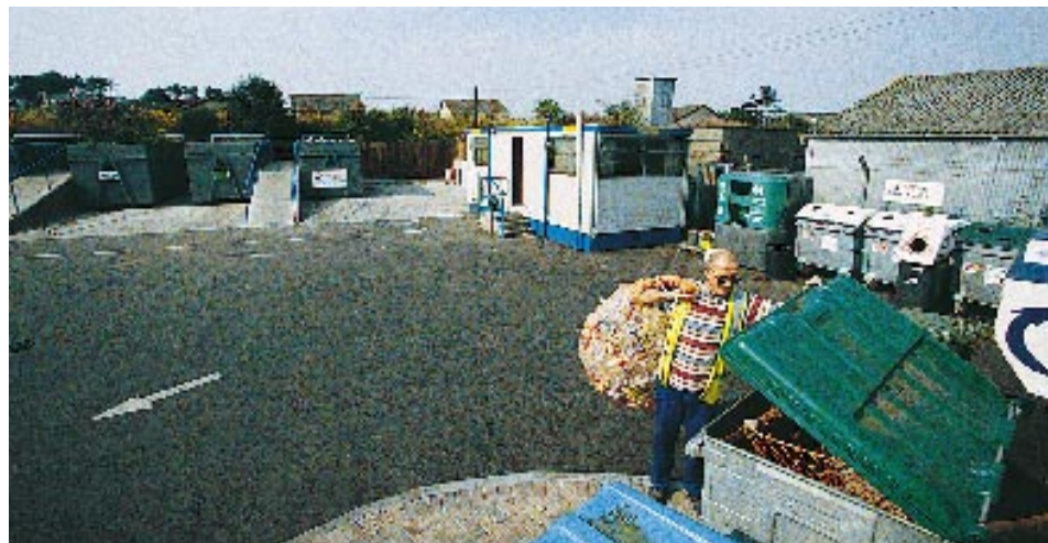
The new recycling facility at Monifieth
