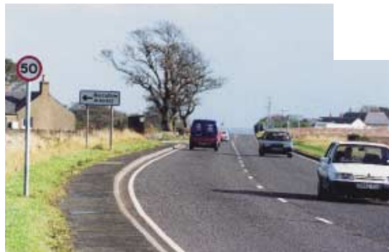
Restricting speed on the A92
