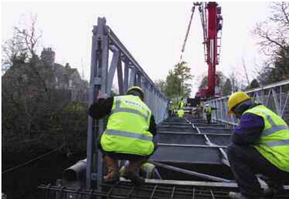
New bridge at Dunlappie
