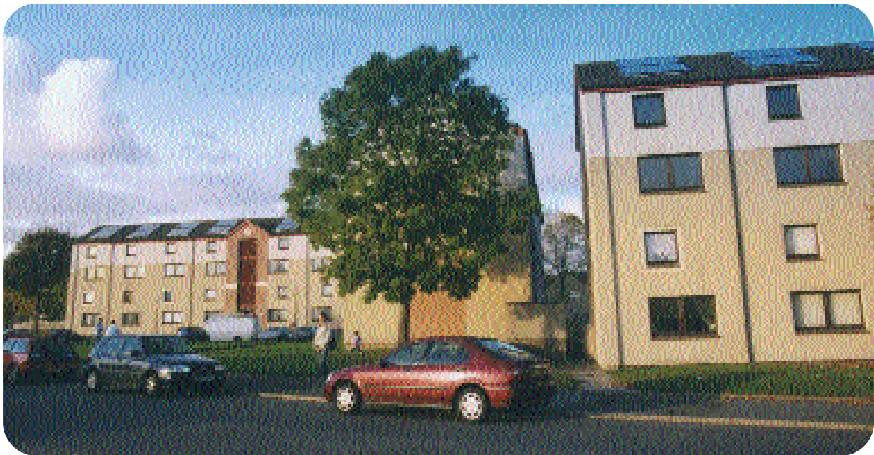
Solar panels in Arbroath
