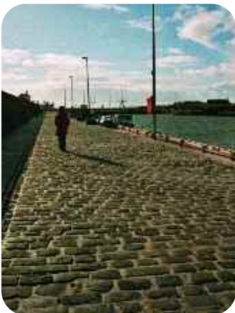
Renewed cobbles at Arbroath harbour
