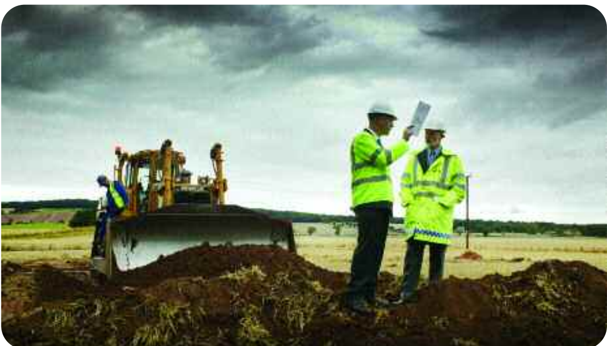
Starting construction of the A92 dual carriageway
