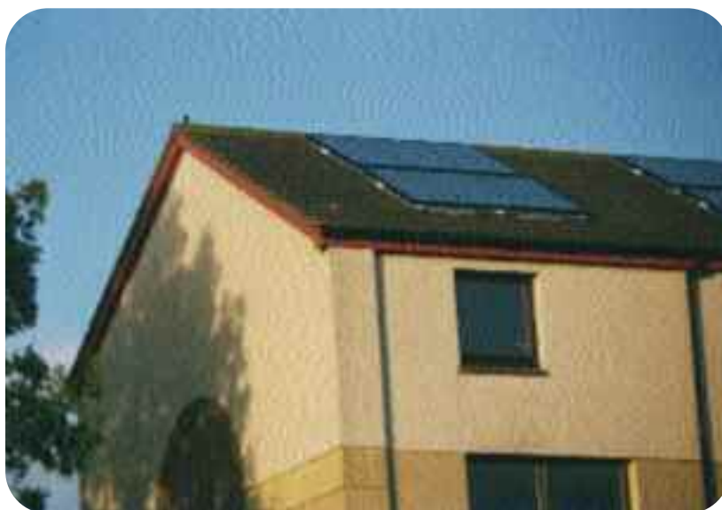
Solar panels in Arbroath
