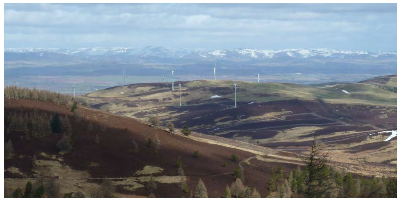
Ark Hill Windfarm
