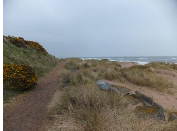
Rock armour covered by accreting dunes in MU1/4
