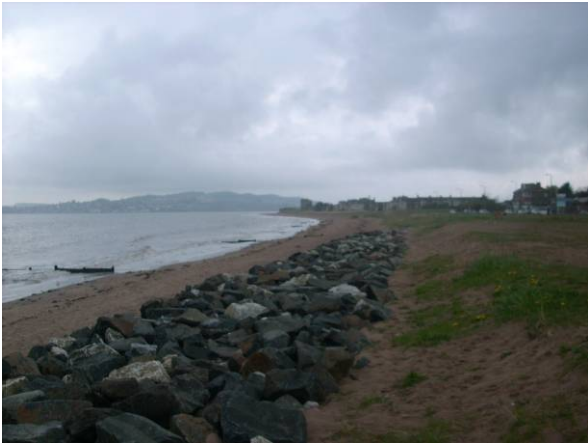
Revetment at Broughty Ferry MU9/4
