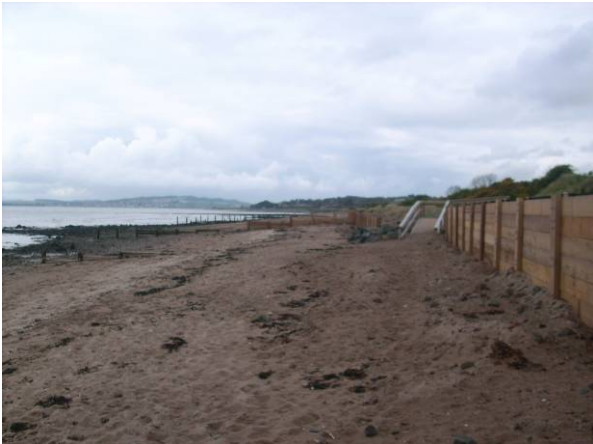
Timber wall and groynes MU9/2
