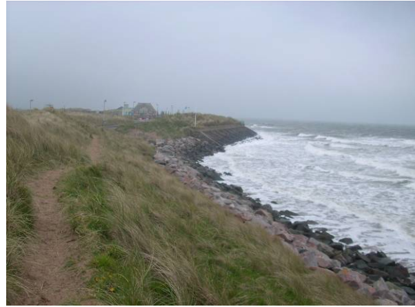
Erosion protection in MU1/3b
