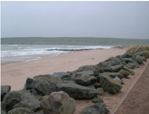
Erosion protection in MU1/3b
