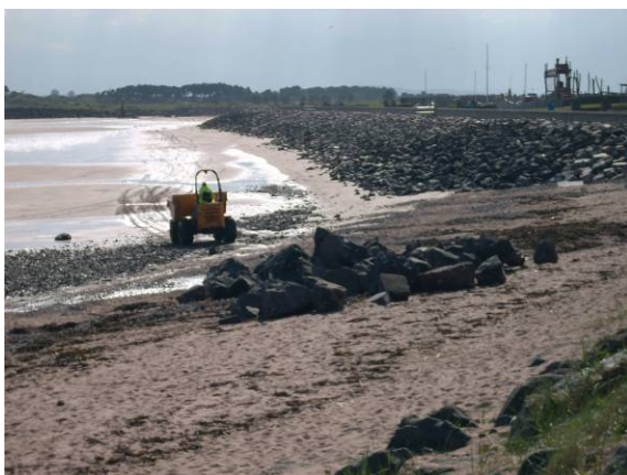
Start of rock armour at transition from MU7/1 to MU/72
