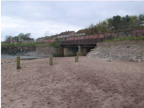
Revetment at Dighty Water outfall, Barnhill MU9/3
