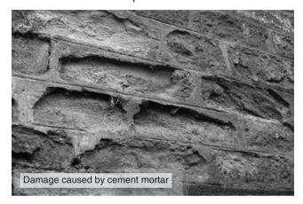
Cement mortar facing and pointing can make a wall less thermally efficient than one built with lime mortar only because water can be trapped rather than evaporating away. Water is an efficient conductor of heat so prolonged wetting of mass walls covered in cement mortar will reduce the thermal efficiency of the building.
