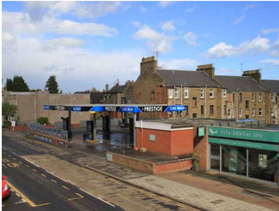
EXISTING FILLING STATION SITE
