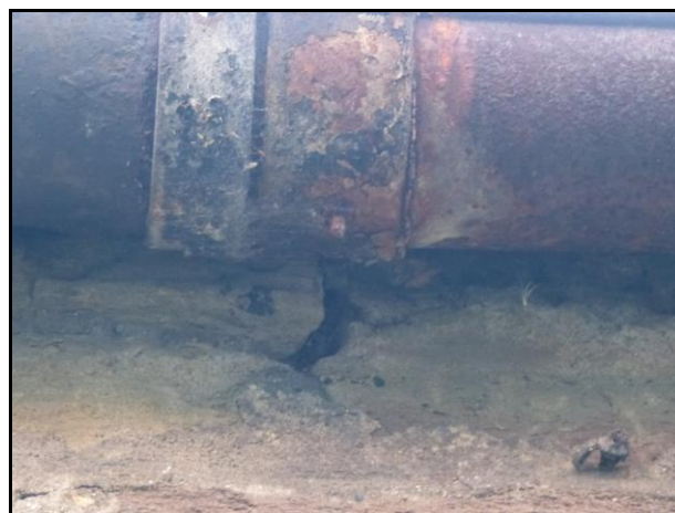
Holes in stonework at wallhead
