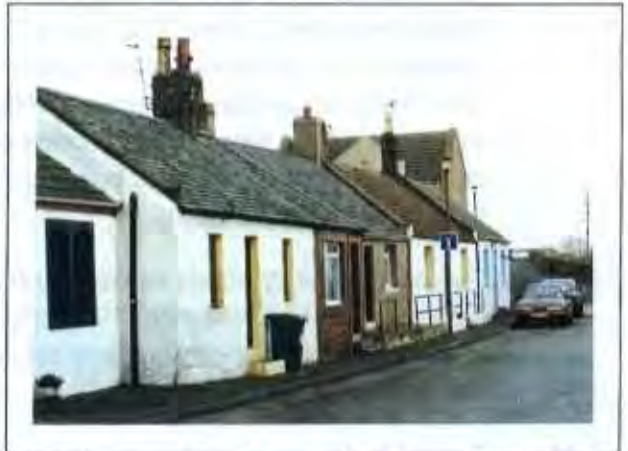
At villages such as Auchmithie, simple working houses were constructed from sandstone and slate, sometimes limewashed.
