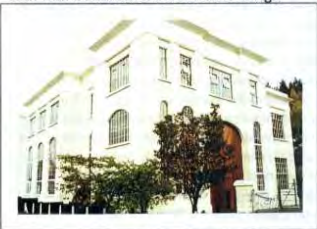
Hydroelectric power has left its mark in the form of dams, enlarged lochs, pipelines, turbine houses (as here on Loch Rannoch) and pylons.
