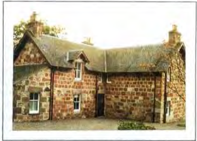
A mixture of pink and grey granite blockwork in this Highland farmhouse.
