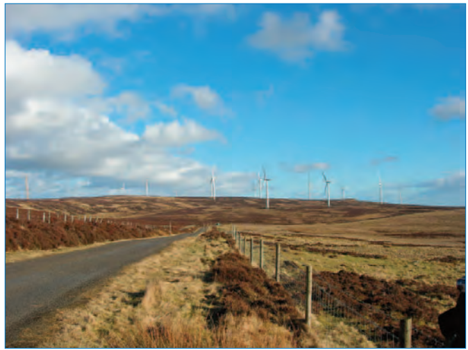
Windfarm relates well to the scale of the landform and the skyline
