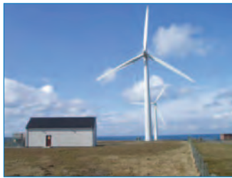
Small windfarm substation
