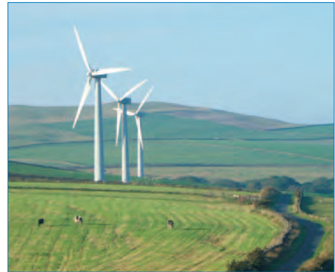
Single line of wind turbines. These possess a visual relationship to each other as well as to the landscape.
