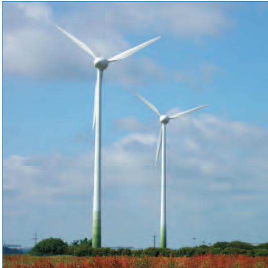
Variable colouring of turbine bases typically does not correspond with the skyline from most viewpoints and increases contrast when seen against the sky. From some viewpoints, this effect can also make the turbines seem to 'float' above the land.
