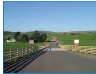
Junction of windfarm access track and public road
