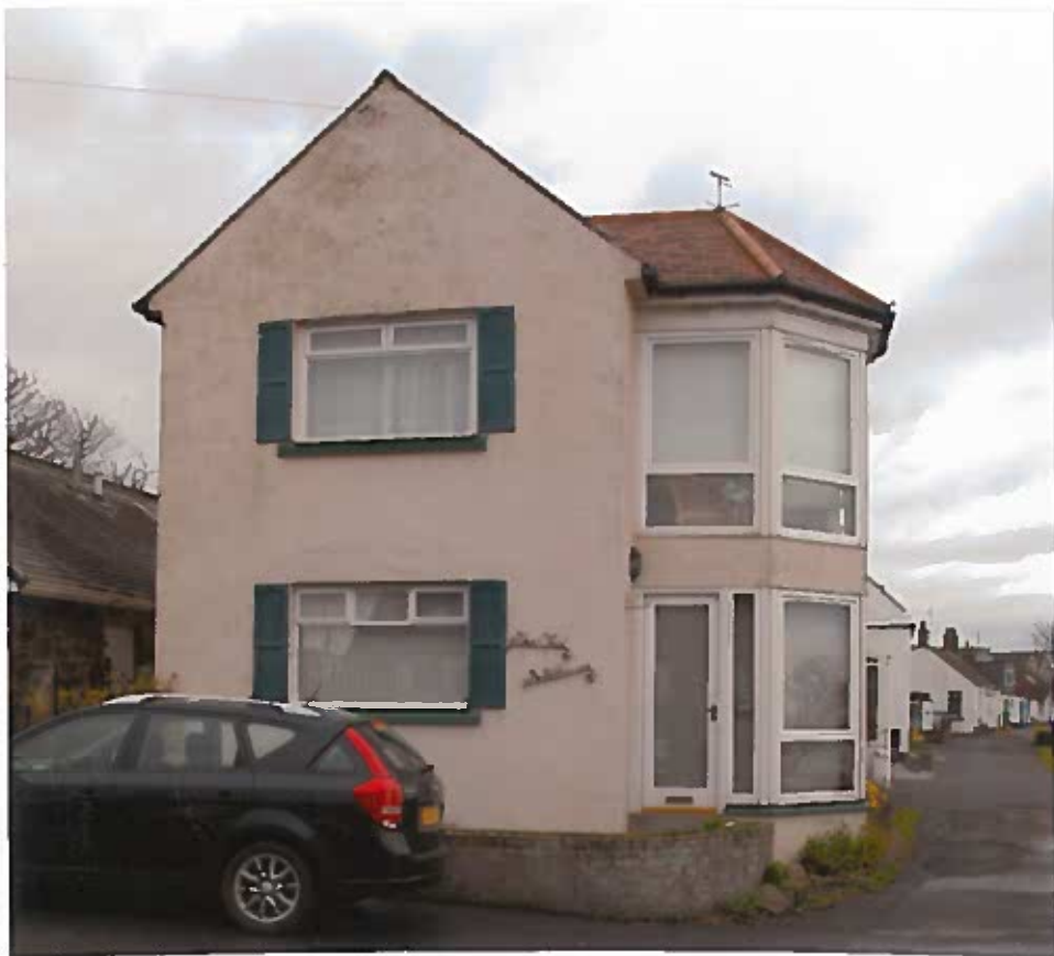
Photograph 10 Two Storey Front extension to Old Boat House at end of East Row
