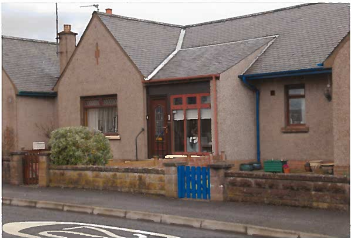
Front Extension to 6 Norries Rd. Only one of twelve house in the area all the same type with an extension.
