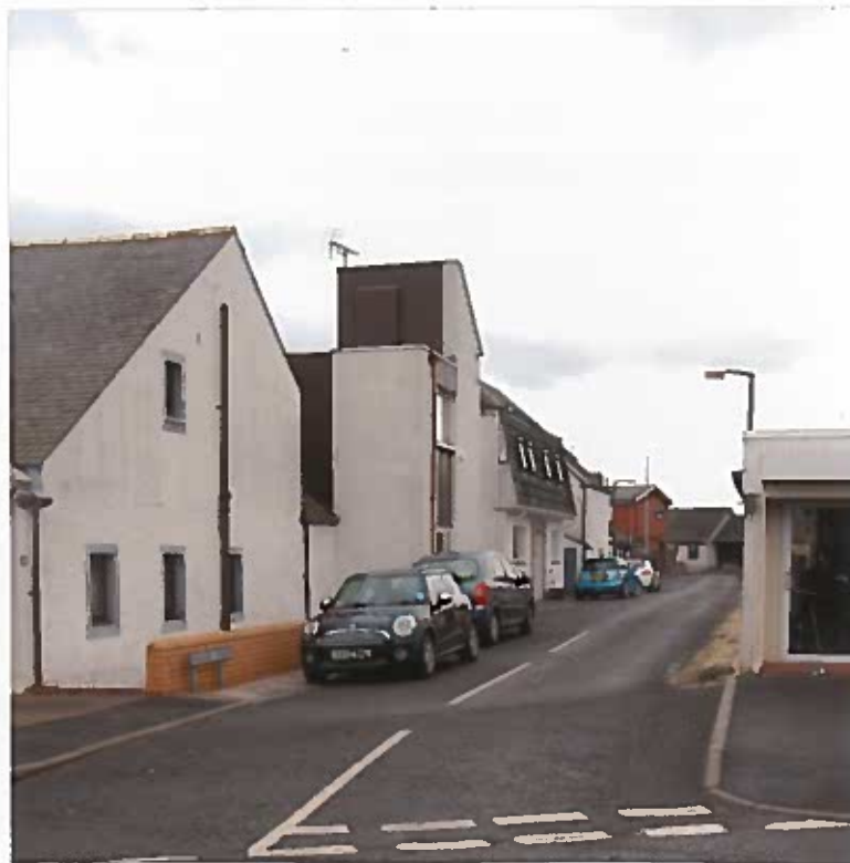
Photograph 2 Mariner St. looking east to west
