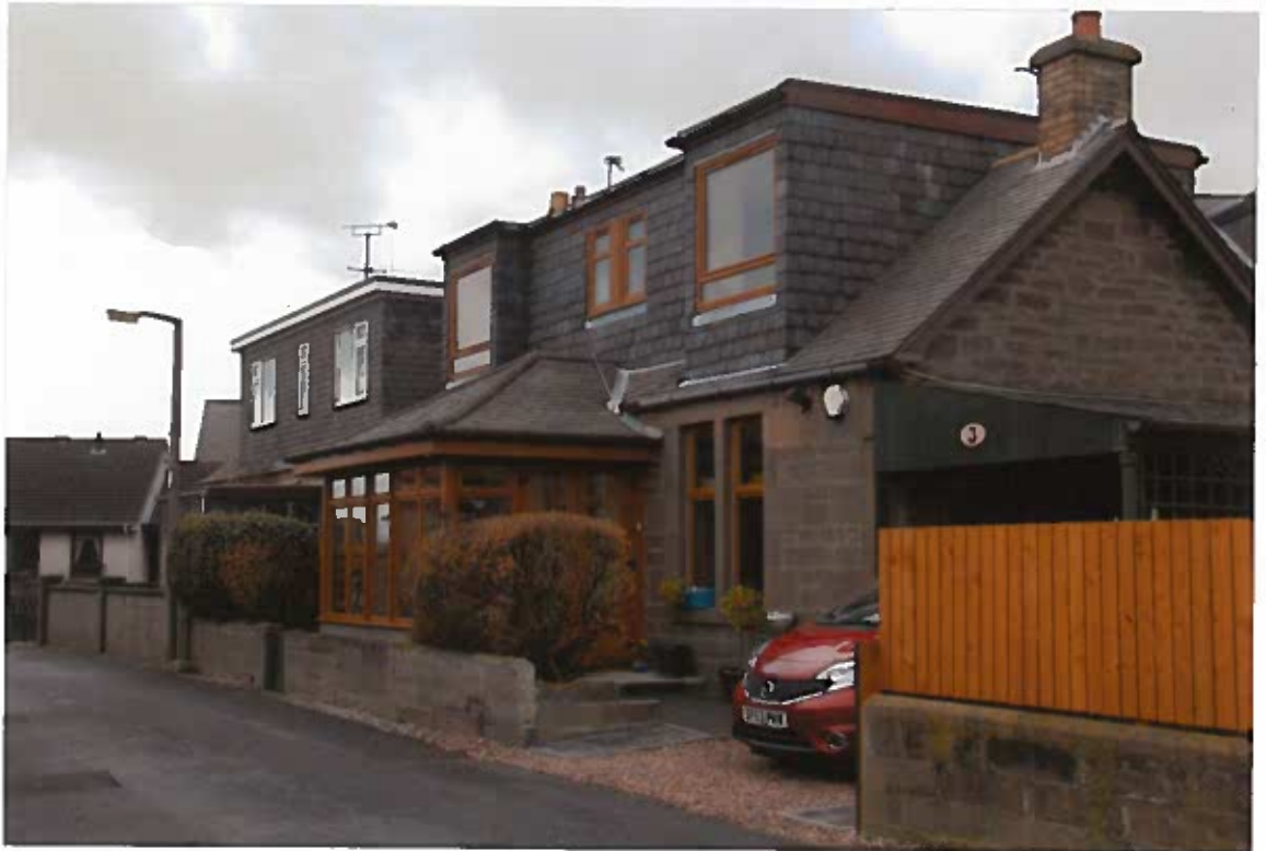
Photograph 8 Front Extension to No 3 Mariner St.
