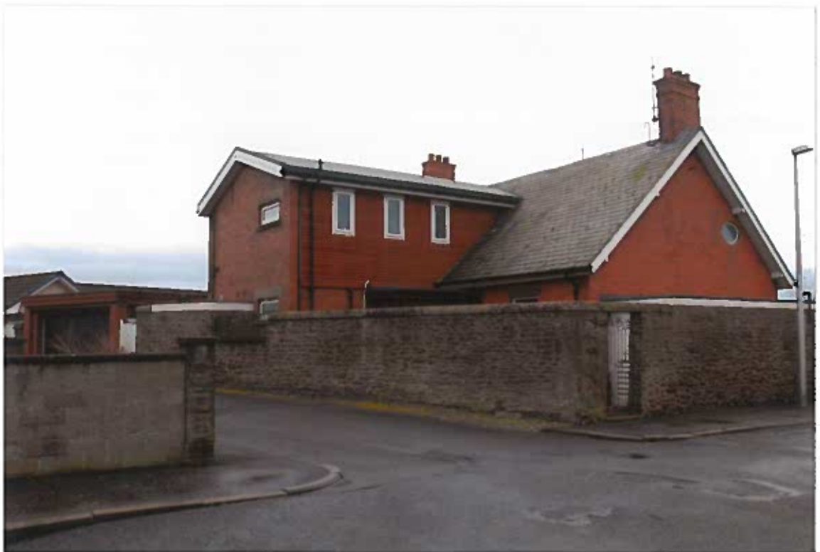
Photograph 4 West veiw of No2 Mariner St., showing extent of extension
