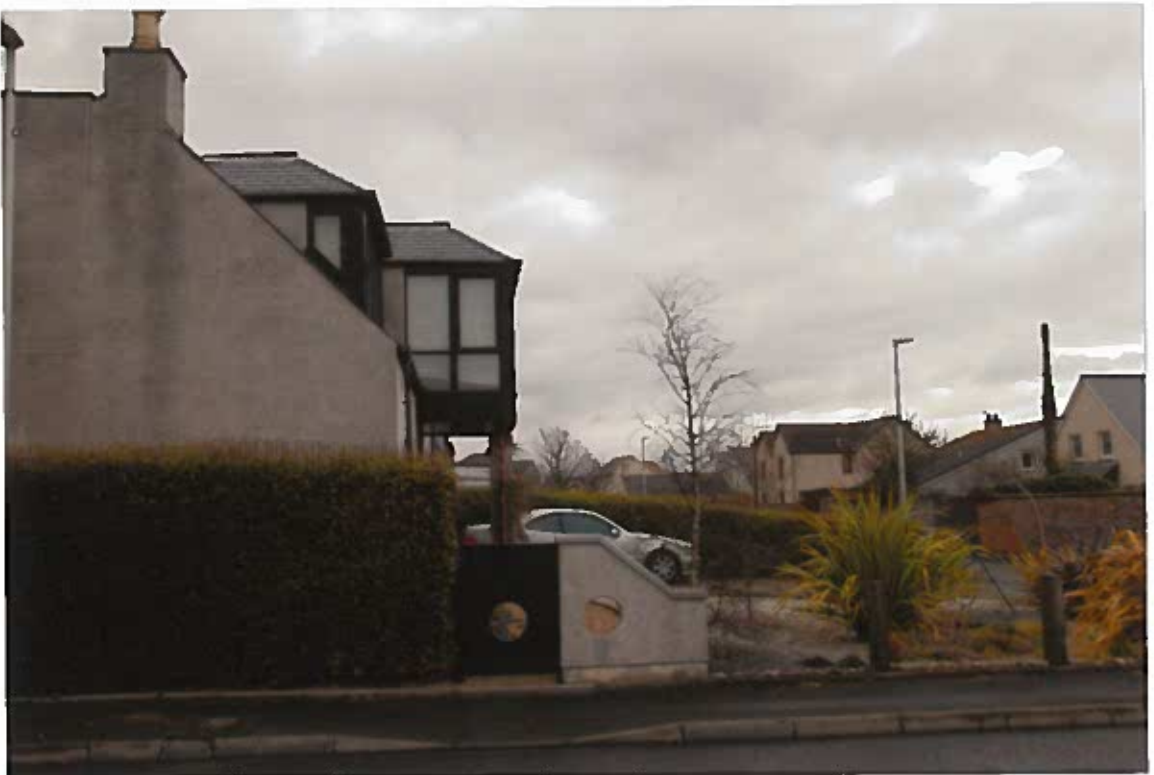
Photograph 5 Front extension to No 1 Long Row
