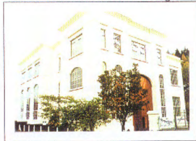
Hydroelectric power has left its mark in the form of dams, enlarged lochs, pipelines, turbine houses (as here on Loch Rannoch) and pylons.
