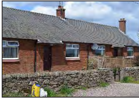
Property 1&2 South-East elevation
