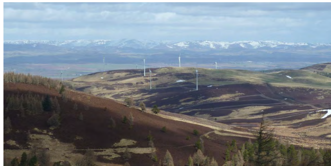
Ark Hill Windfarm
