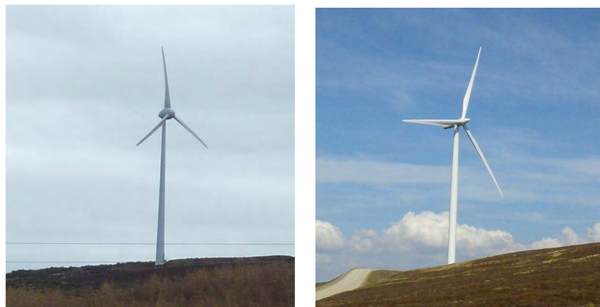
Enercon and Siemens turbines have different nacelles, blades and towers leading to significant differences in appearance
