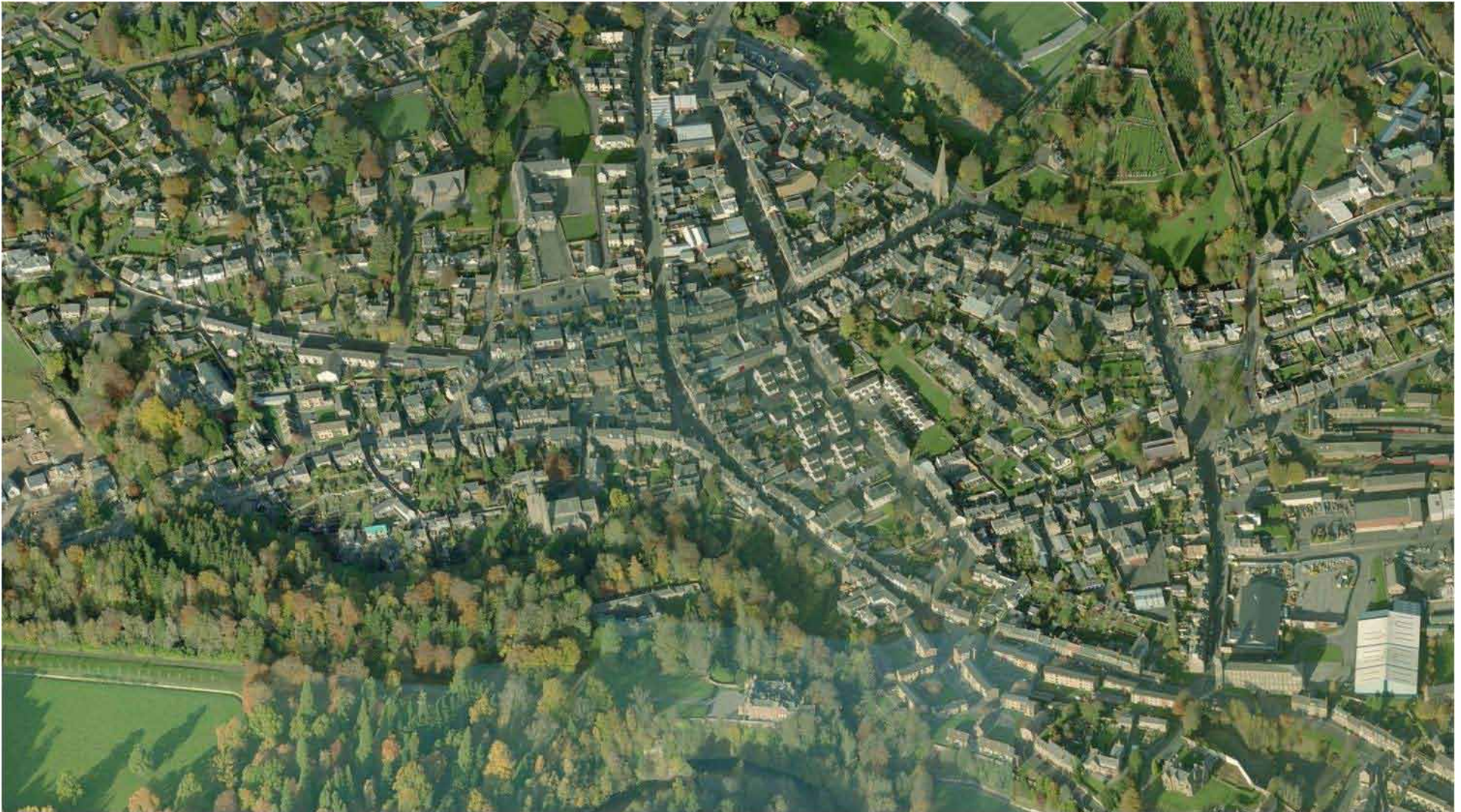
Aerial Image of Brechin
