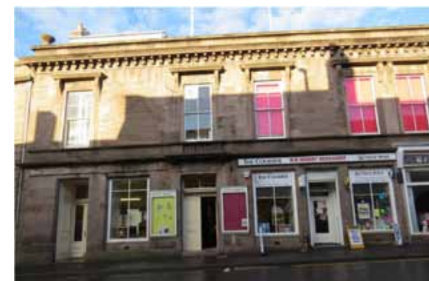
Town Hall Exterior
