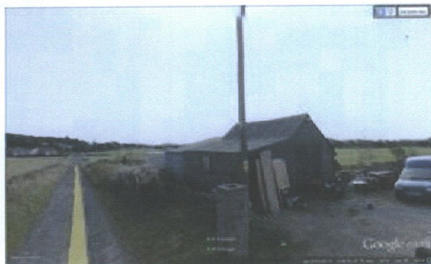
Fig 4: The joiner's workshop will be demolished.
