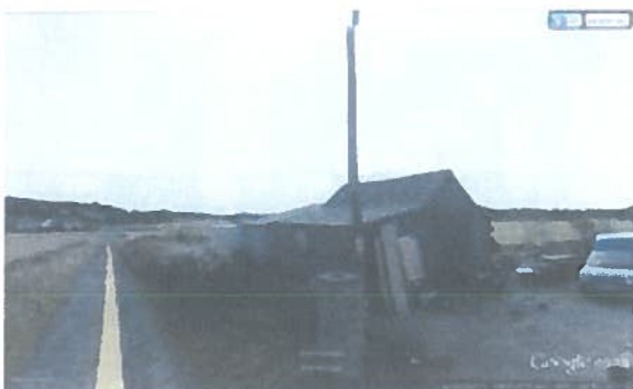
Fig 4: The joiner's workshop will be demolished.
