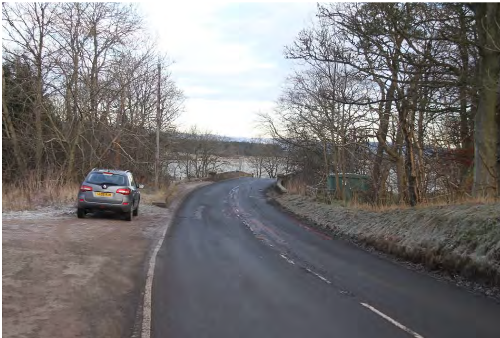
B966 Westwater Bridge looking north
