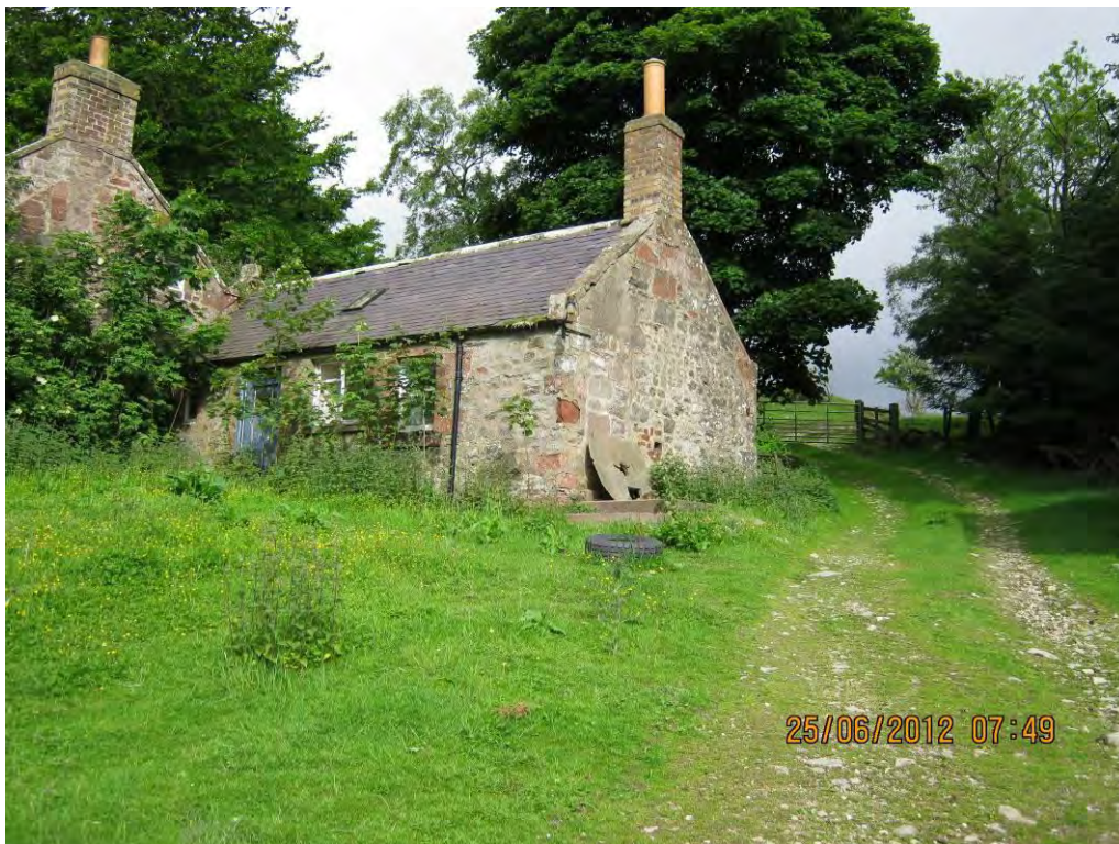
Figure 5.9 View of Abandoned House from South (Bats present in both buildings)
