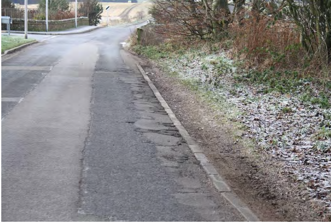
Lethnot Road in Edzell - north side of carriageway
