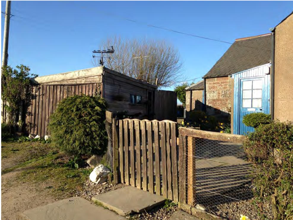
Tillydovie Cottage. Note how views are obscured by tenant's sheds.
