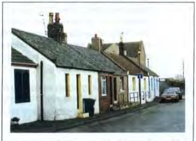
At villages such as Auchmithie, simple working houses were constructed from sandstone and slate, sometimes limewashed.
