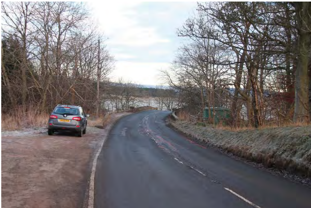
B966 Westwater Bridge looking north
