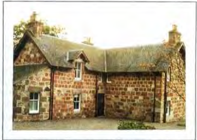
A mixture of pink and grey granite blockwork in this Highland farmhouse.
