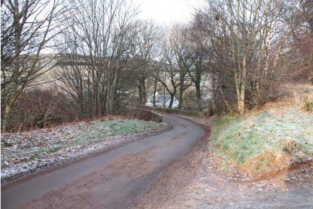
Bridge of Margie looking west
