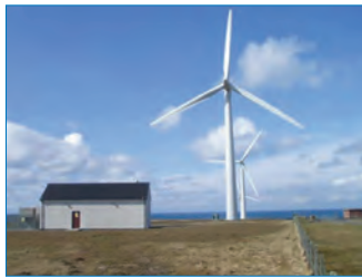
Small windfarm substation
