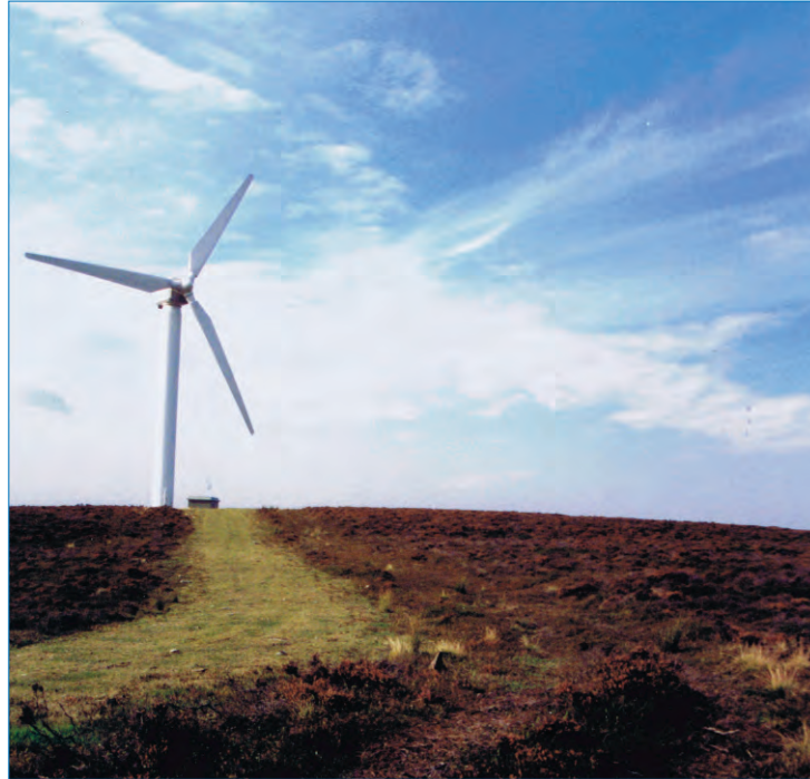
Partial restoration of access tracks to grass
