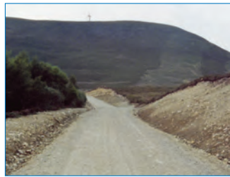
Windfarm access track across slopes
