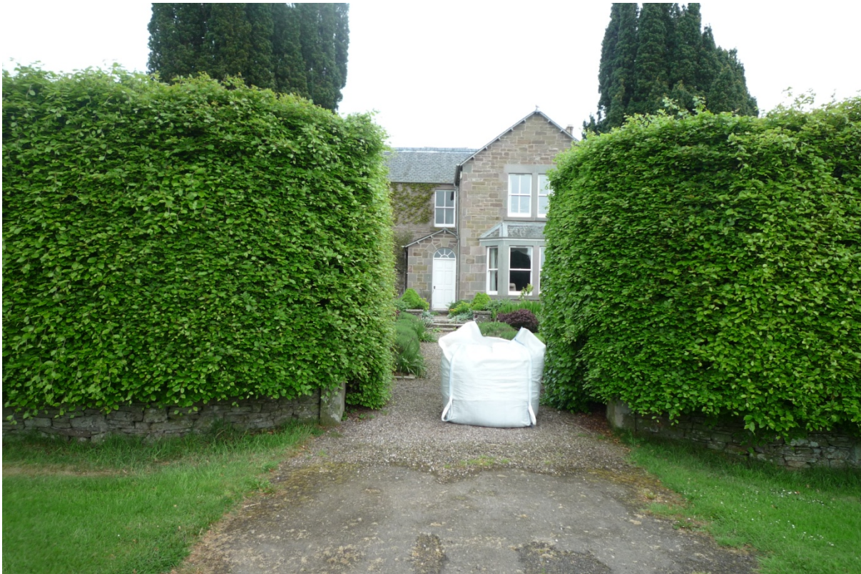
Figure 2: Gask Farmhouse. Taken facing east. The property is well-screened by surrounding established hedgerows. Large agricultural buildings also lie to the west of the Farmhouse, further screening the property from the appeal site. Please note there was no objection from this property.
