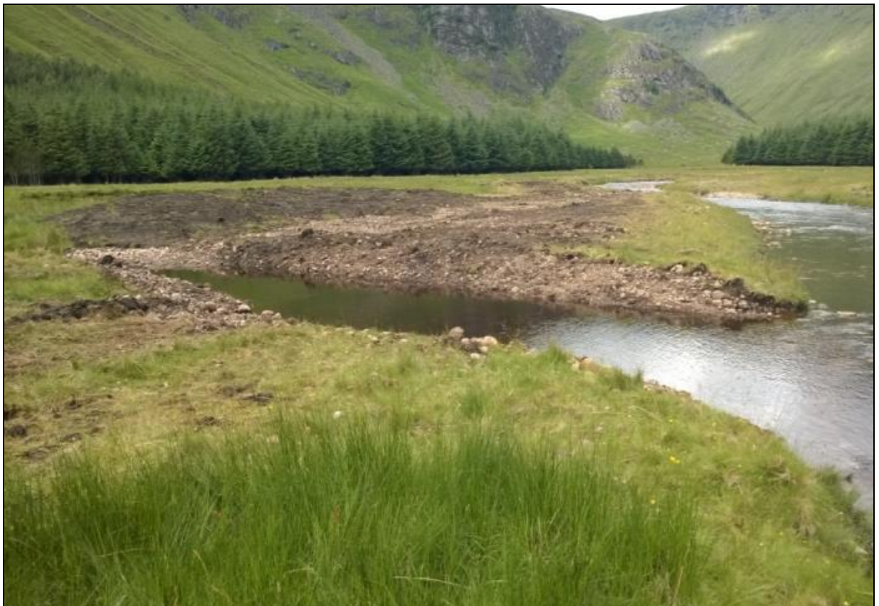
Acharn – removal of rock armour bank protection
