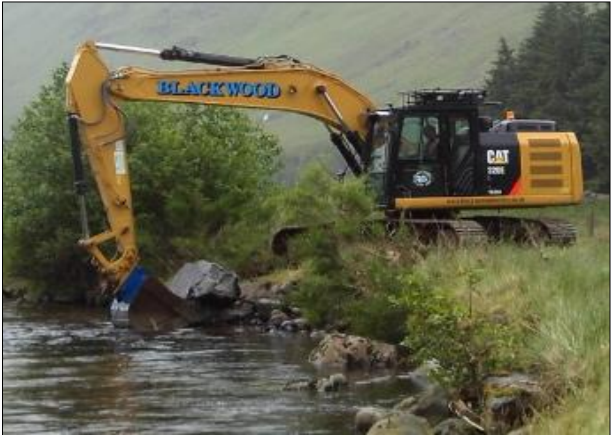
Acharn – removal of rock armour bank protection
