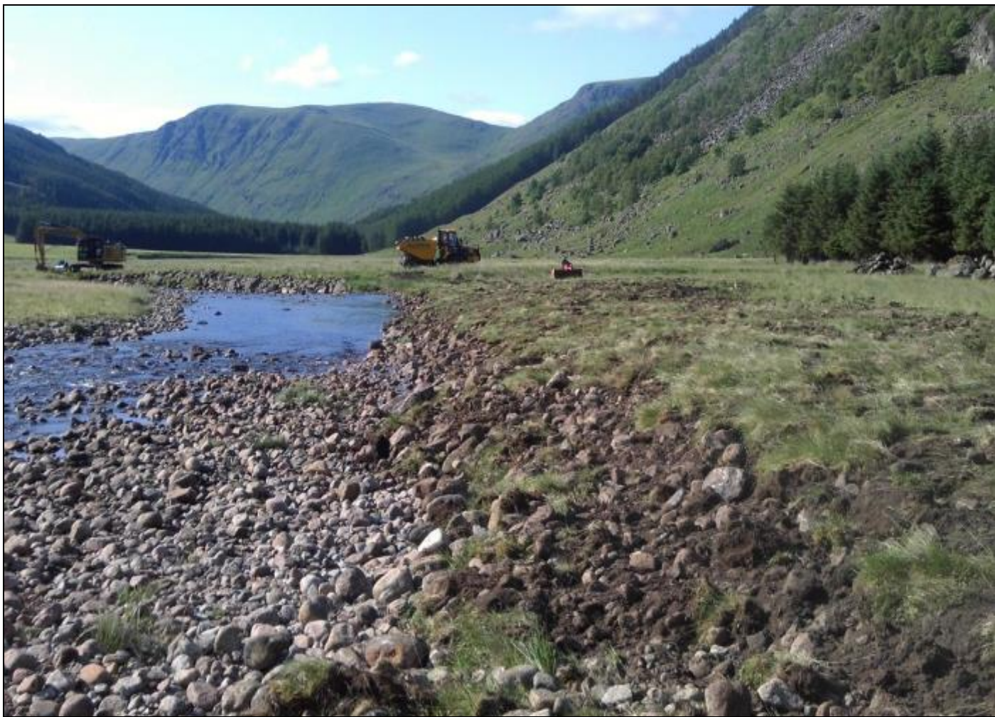
Re-profiled bank at Moulzie immediately after removal of boulder bank protection
