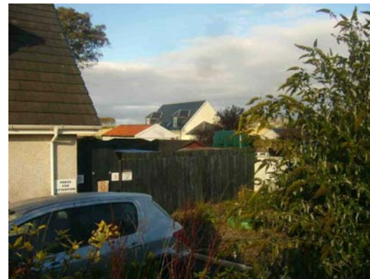
Existing backland development in Marywell.
