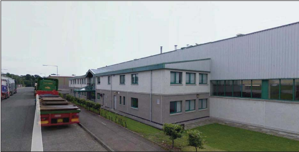
The north-western façade of the building showing the commercial offices.
