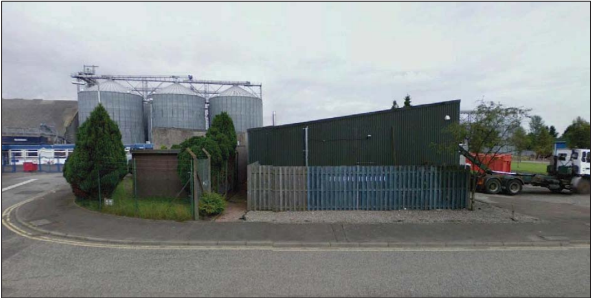
The southern façade of the unit, which faces the turbine.
