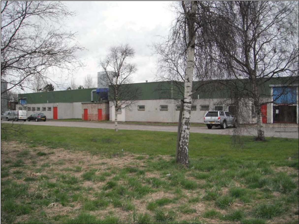
Main façade of industrial units showing potentially affected windows.
