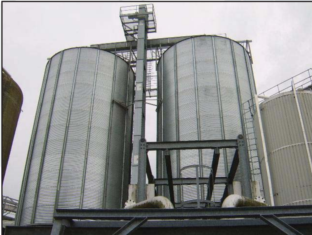
Figures 3 & 4. Area near turbine location
