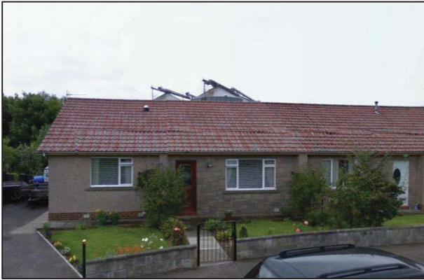
The northern façade of the property facing away from the turbine
