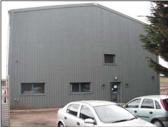
North-western façade of the property facing obliquely away from the turbine.
