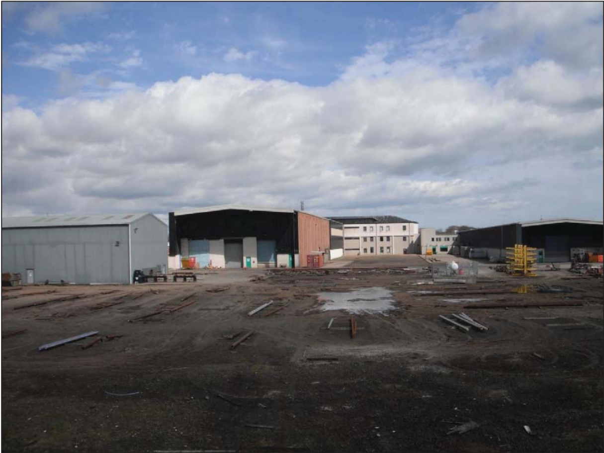
South-western façade of the building. The offices are visible in the distance, between the two large warehouses.
