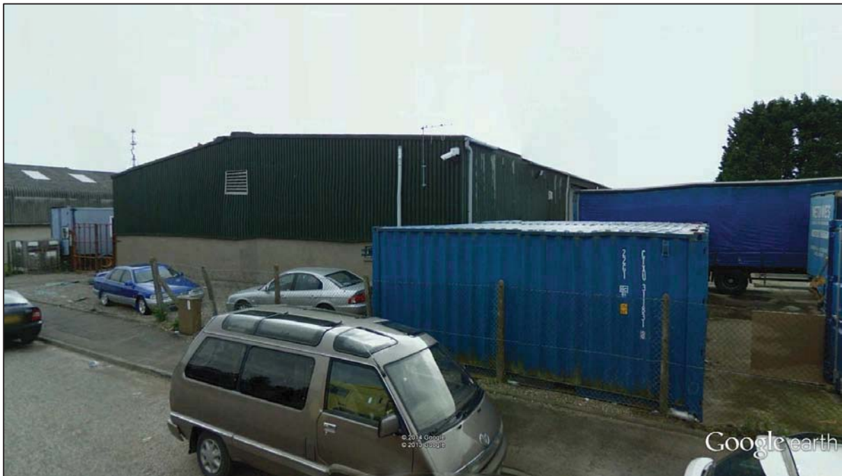
Photograph of the northern façade of the property. Western façade is to the right of the picture
