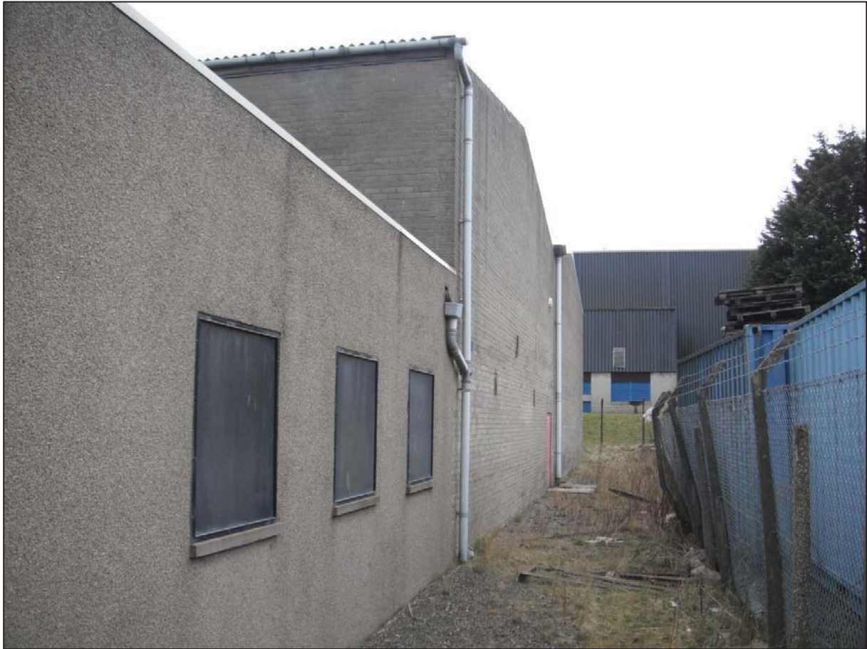
South-western façade of the premises, oblique to the turbine
