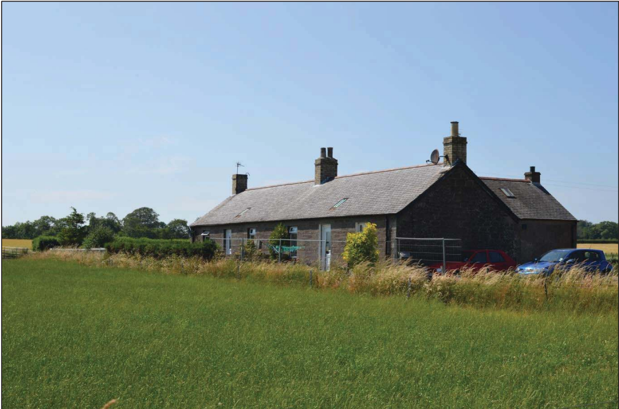
South-eastern façade of the properties, which face the turbine
