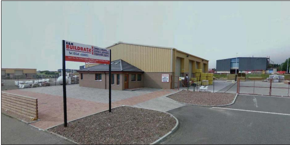
The north-eastern façade of the building, facing away from the turbine
