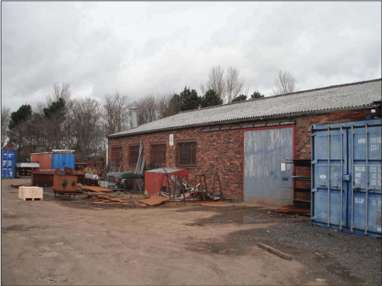
South-western façade of the Smithy premises which is oblique to the turbine.
