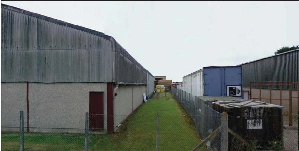
South-western façade of the building which faces the turbine
