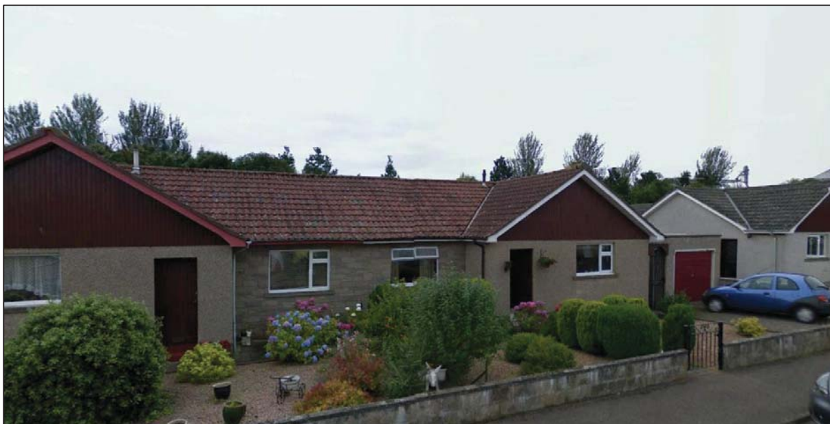
The northern façade of the house, which faces away from the turbine. Shelter belt of trees visible to the rear.
