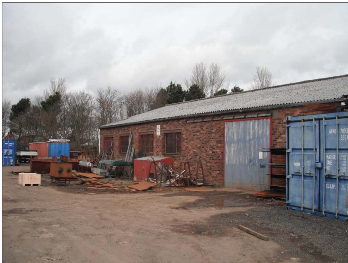
South-western façade of the Smithy premises which is oblique to the turbine.
