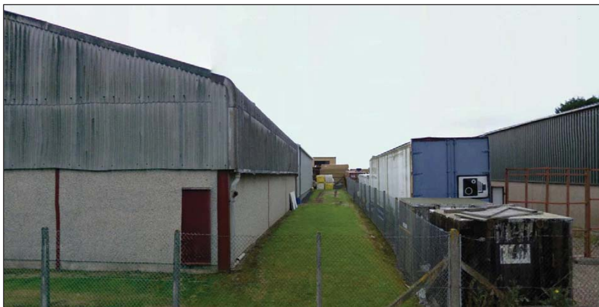
South-western façade of the building which faces the turbine
