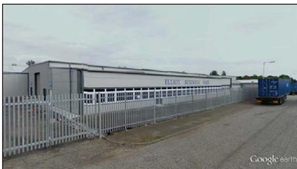
Southern portion of the south-eastern façade of the Business Park offices
