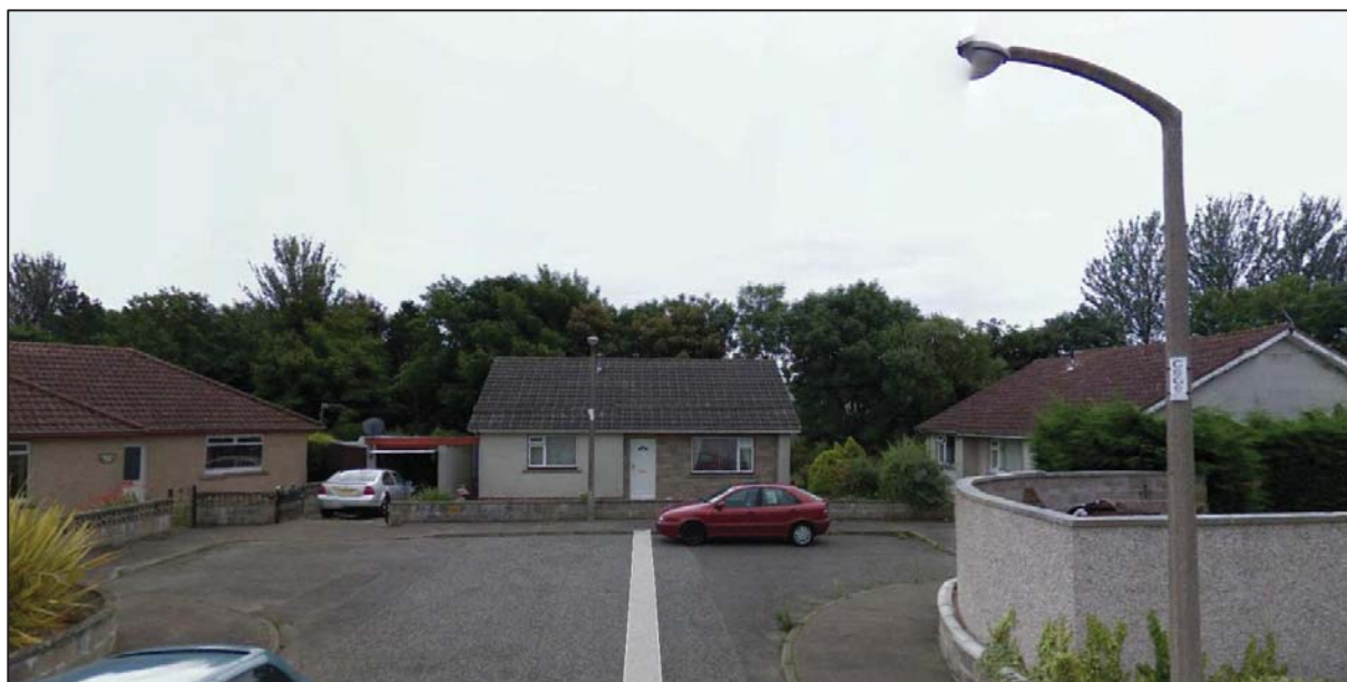
The northern façade of the house, which faces away from the turbine. Shelter belt of trees visible to the rear.
