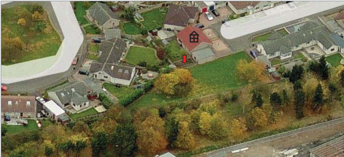
Figure 8.4: Satellite image including H2 at Patrick Allan Fraser Street.
