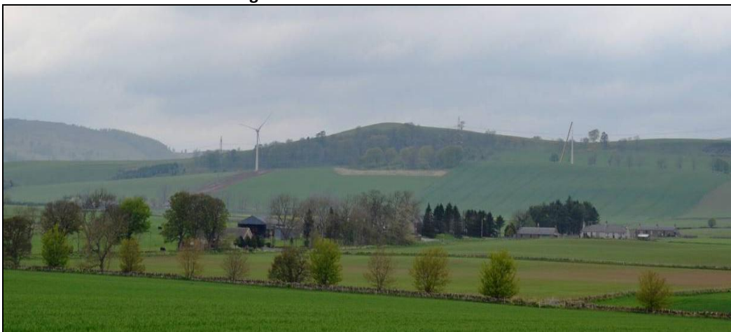
Figure 6 – Turbines (under construction) near Memus
