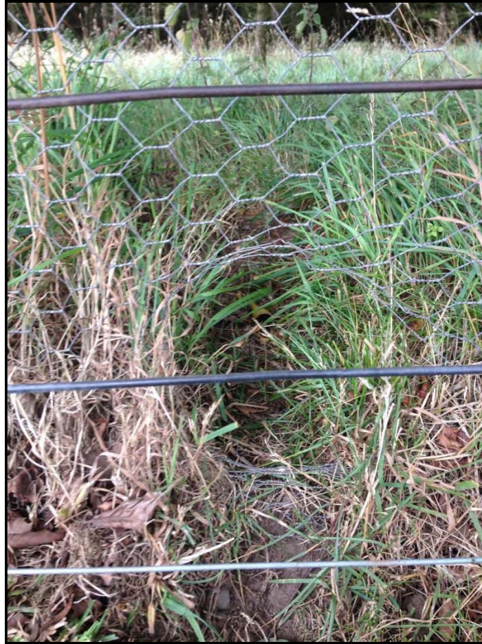
Photograph 3: A breach in the deer fence along the east site boundary.
