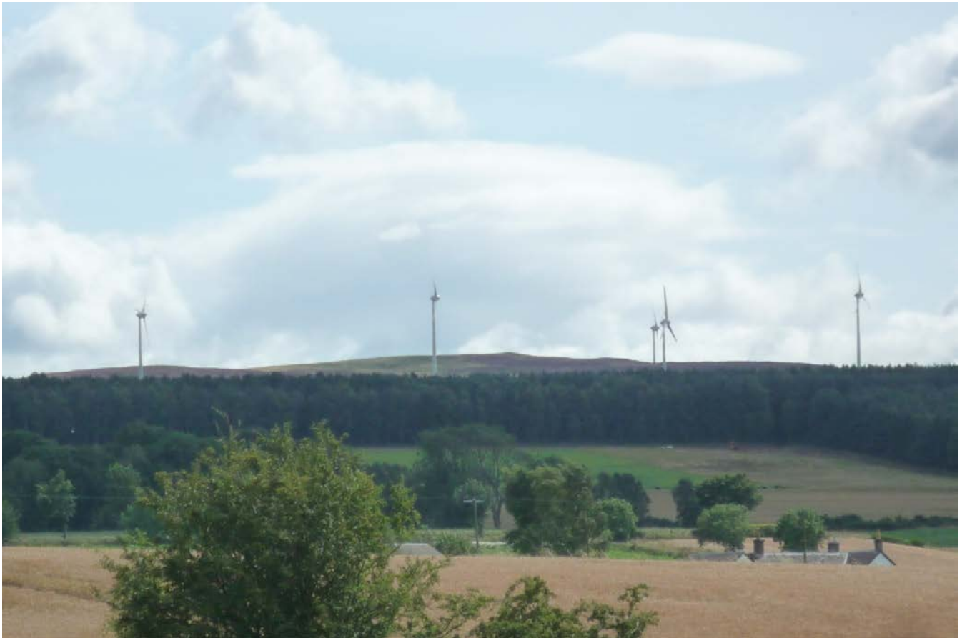
Figure 3: Ark Hill windfarm from A94
