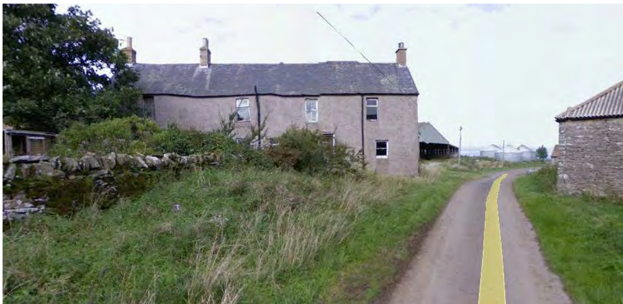
Figure 13: View of Unnamed Property (~700m from turbine) looking north-north-east along public road. It shows that the majority of windows are orientated to the south-east (i.e. away from the turbine). A small garden lies to the south-east of the dwelling. To the north-west (i.e. towards the turbine) views are obscured by very close substantial farm buildings and rising ground.
