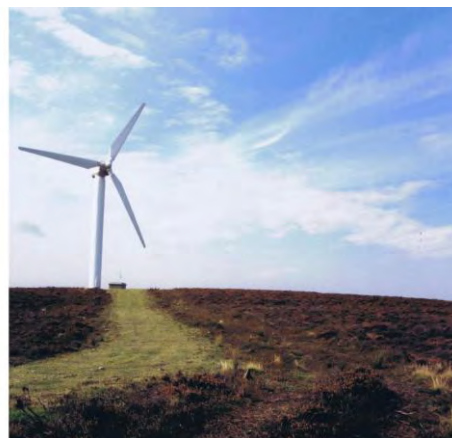
Partial restoration of access tracks to grass
