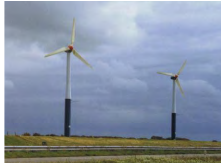
Different colour of wind turbine components creates a more complex image and means the visibility of different sections varies
