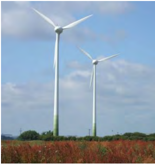
Variable colouring of turbine bases typically does not correspond with the skyline from most viewpoints and increases contrast when seen against the sky. From some viewpoints, this effect can also make the turbines seem to 'float'
