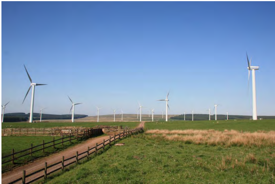
The turbines used in wind farm extensions should closely match the existing turbines, such as in this example (original turbines in foreground, new turbines in background)
