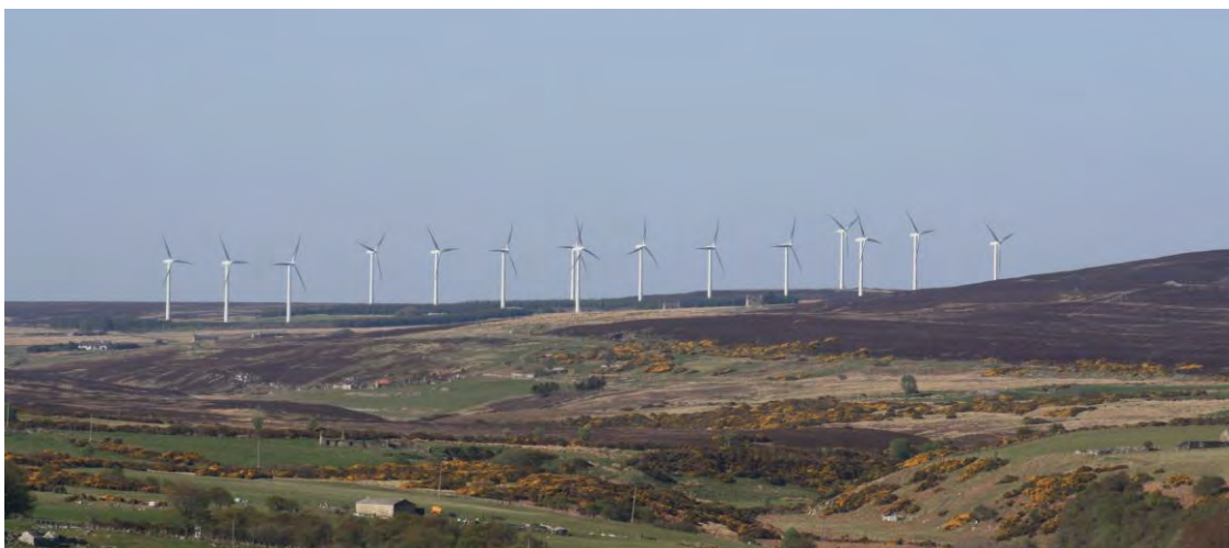
Regular layouts require careful assessment from key viewpoints and care is required during micrositing
