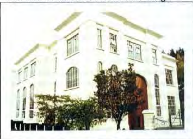
Hydroelectric power has left its mark in the form of dams, enlarged lochs, pipelines, turbine houses (as here on Loch Rannoch) and pylons.
