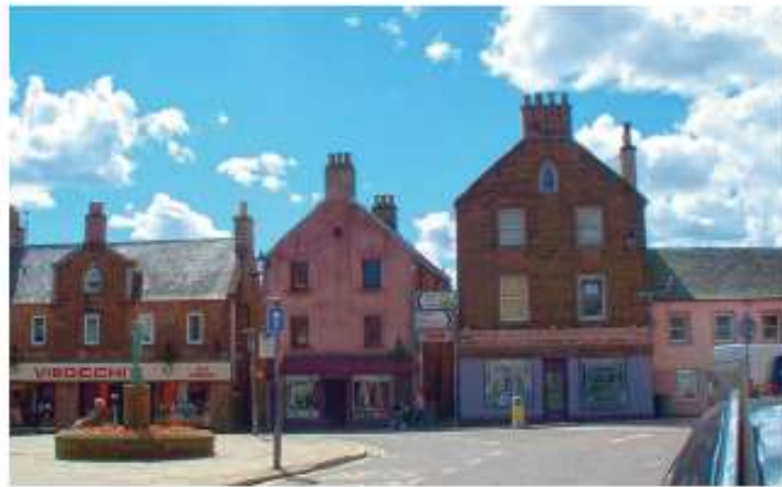
Figure 9 Gable end buildings on High Street
