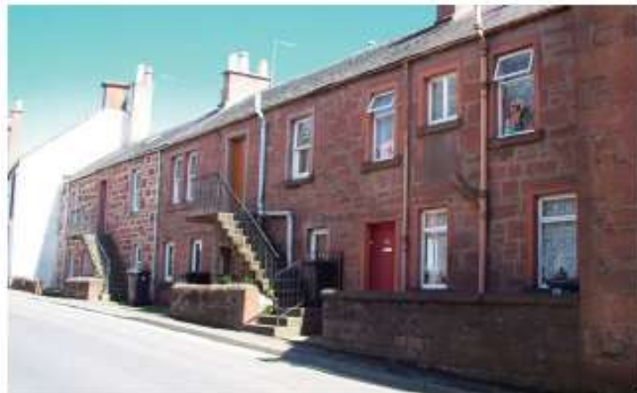
Figure 10 Fore-stairs in St Malcolm's Wynd
