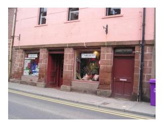
Re-pointing works and new stone indents are proposed on the lower part of the shop window to replace eroded stone. The repair works will not only improve its structural stability but will also result in the improvement of the appearance of this traditional listed building. Additional repair/repainting works are proposed to the timber display windows and entrance door.
