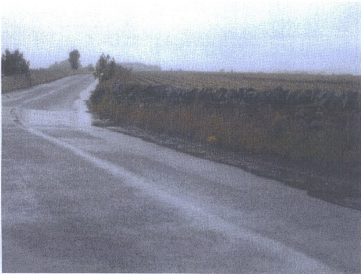
Runoff collecting along south side of proposed site (looking towards Murroes School)
