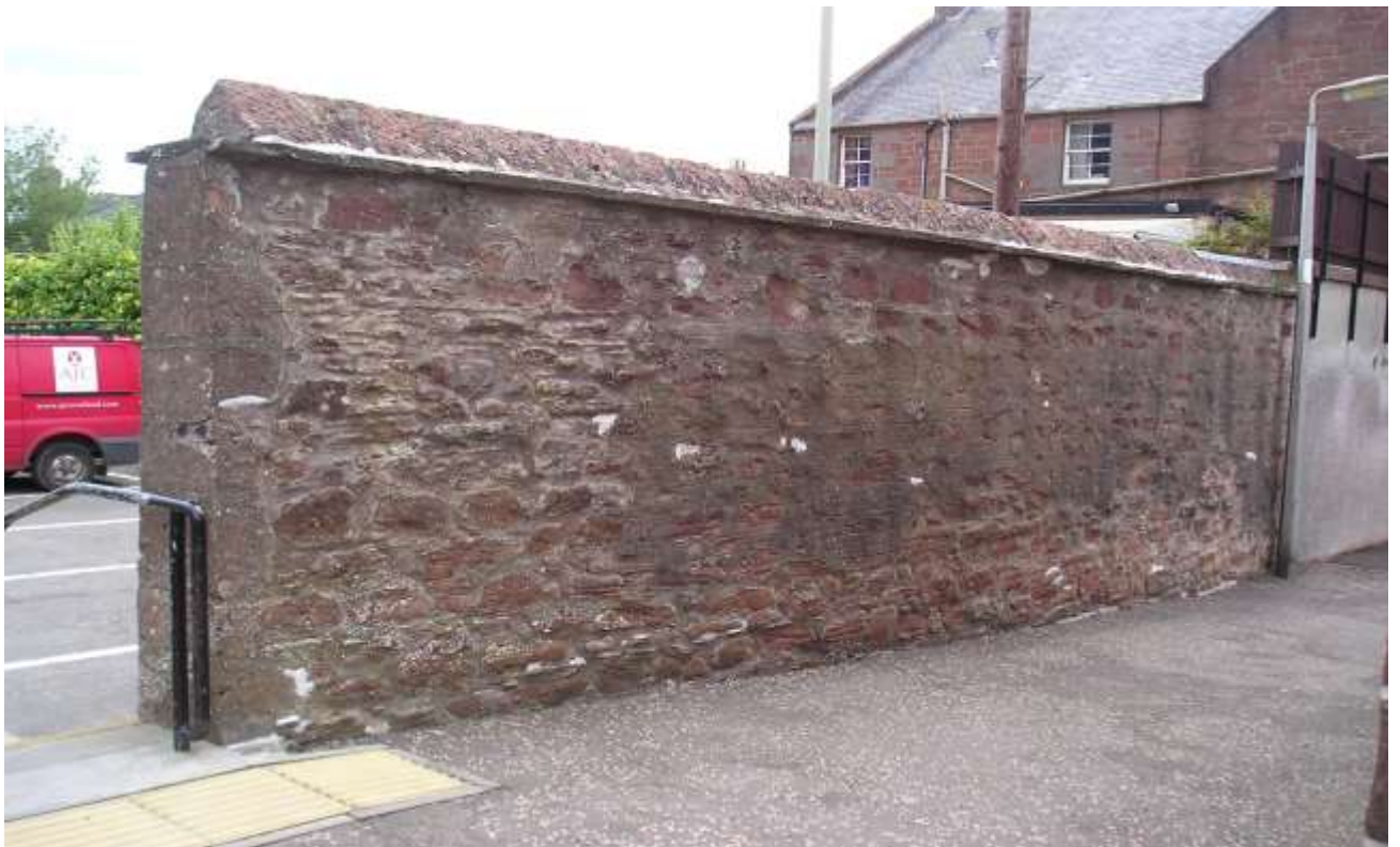
PHOTOS OF THE WALL IN ST. COLME'S CLOSE / JULY 2017
