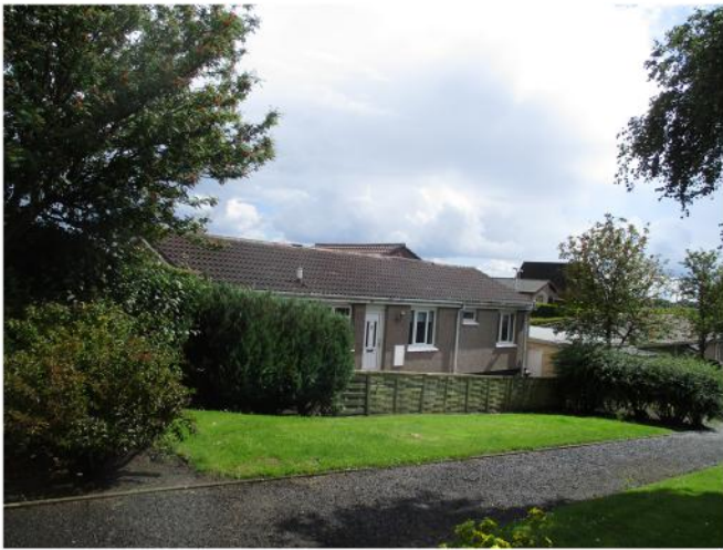
1) Photograph from applicants site showing neighbours extension breaking the ridge line to the front elevation.
