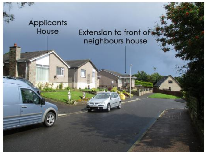
2) Photograph showing precedence set for front extension.
