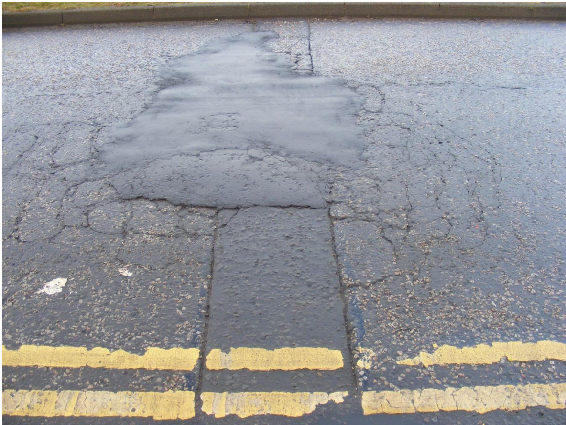
Figure 3 – example of a reinstatement which appears to be having an effect on the surrounding carriageway
