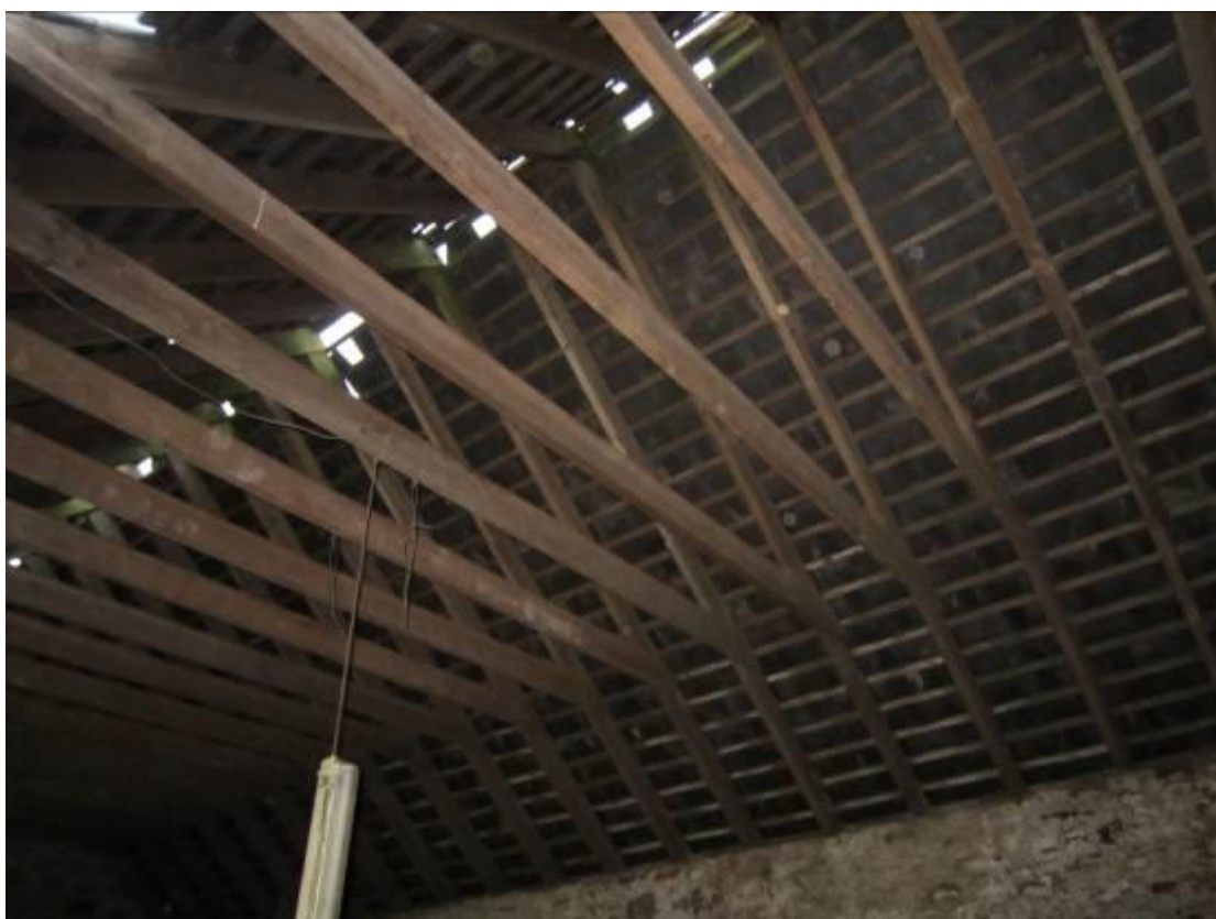
Interior of slate roof
