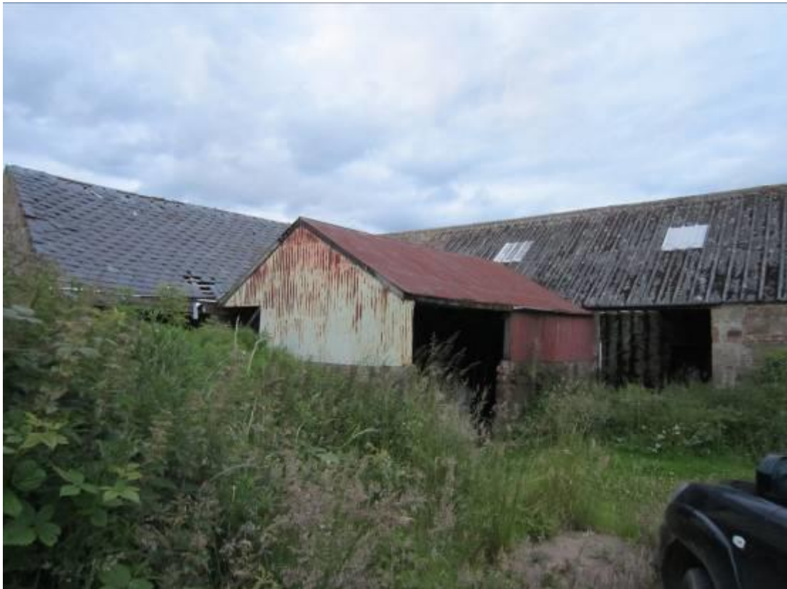
Southeast showing different roof materials
