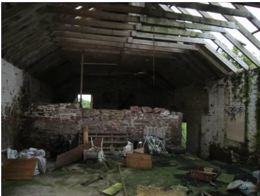
Interior of asbestos roof
