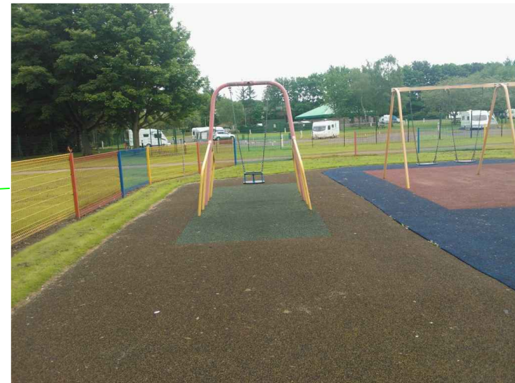
Supply and install 60m of multi coloured, red, yellow green and blue Heavy Duty Roll top fence 1200 mm high supported by matching Twilfix 2000 box section posts. As to Specification. No RT23 or Similar
