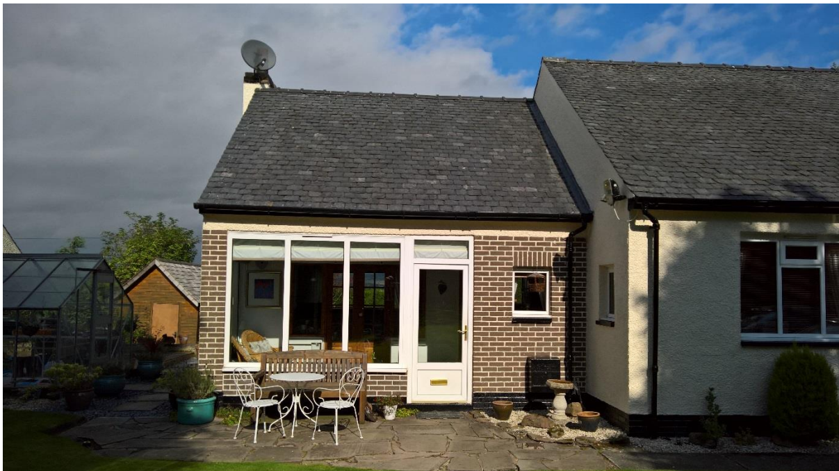
The shading effect of the existing conifers in the garden can be seen here as the shadows cover the south wall of the house and part of the patio.
