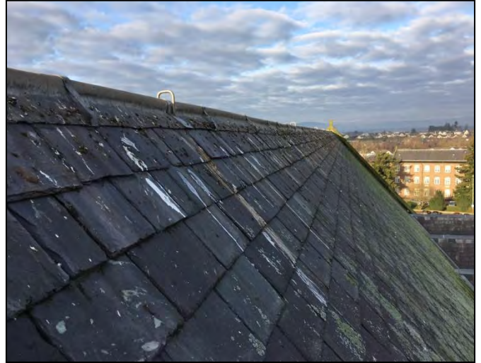
Photo 5: Roof showing flush slates and well sealed ridge
