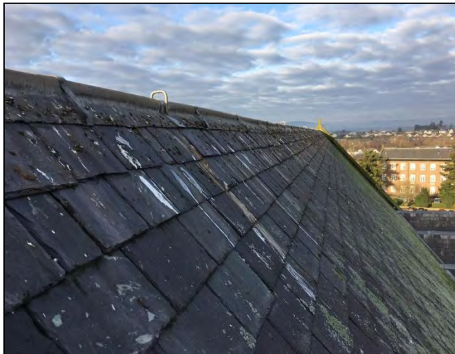
Photo 5: Roof showing flush slates and well sealed ridge
