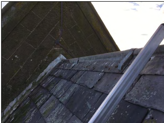
Photo 4: Coping at southern gable blocking access
