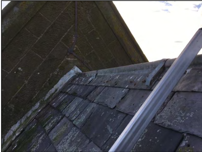
Photo 4: Coping at southern gable blocking access
