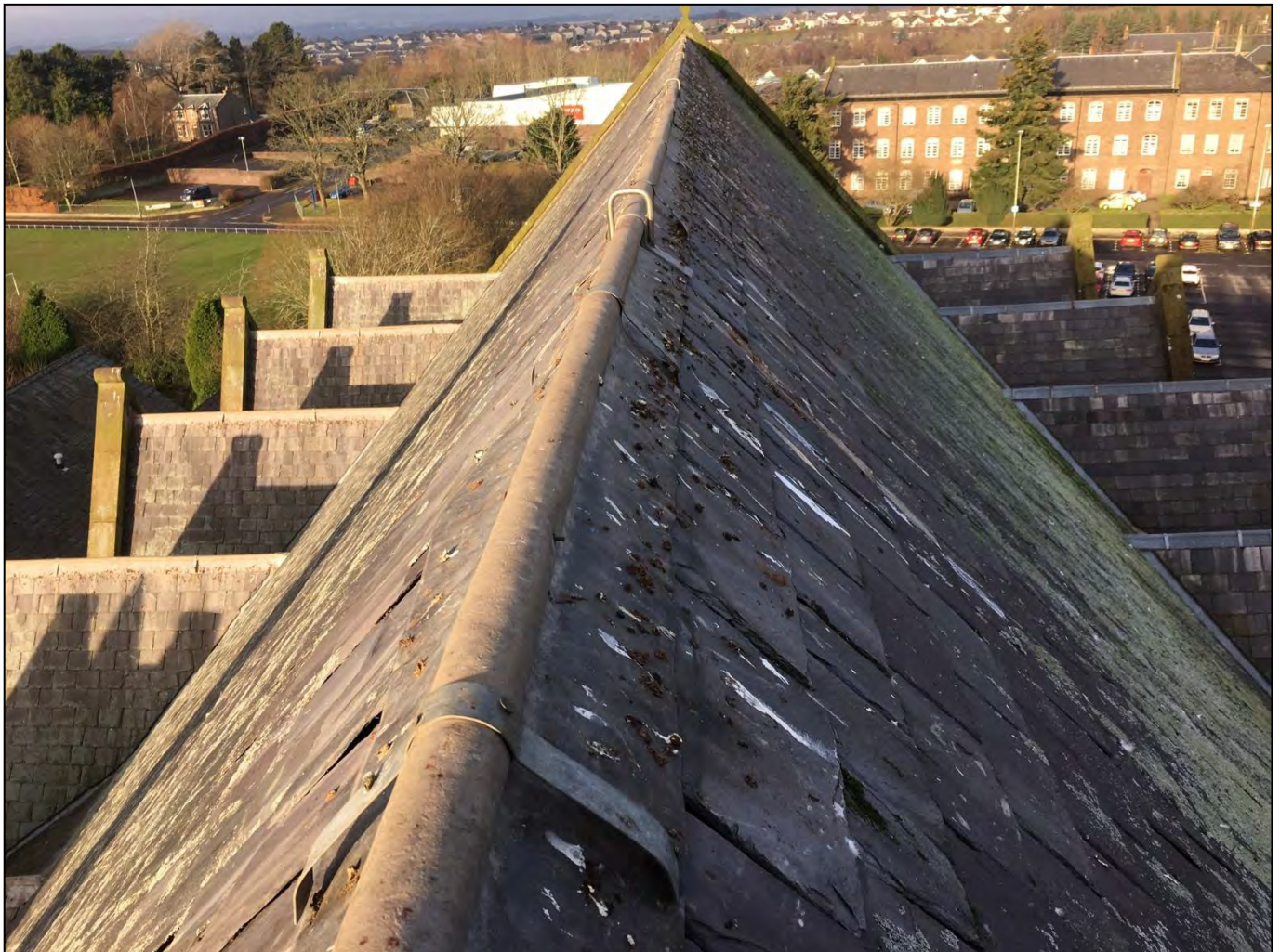
Photo 3: High roof structure (looking north) showing window dormers
