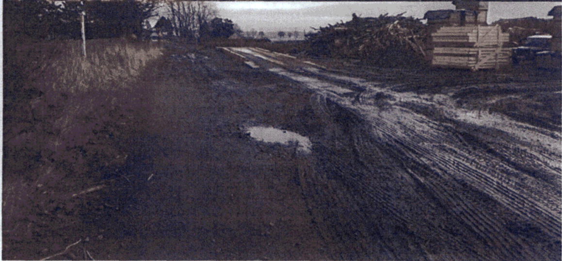
12. Pimperdam Biomass Facility. Lorry damage to surrounding tracks
