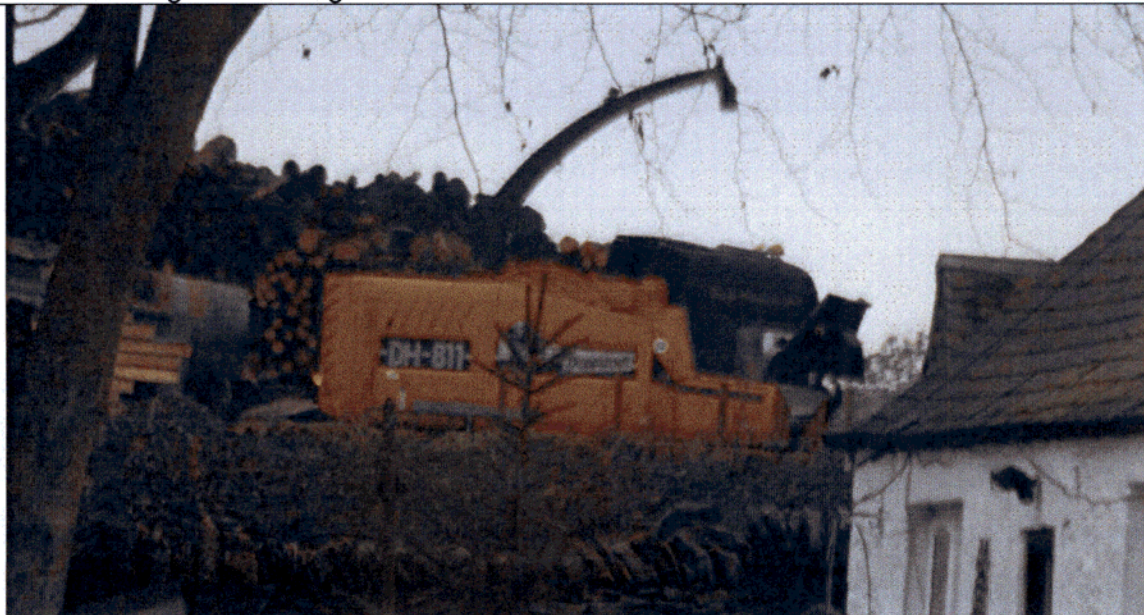
Above: New grinder arriving on site immediately prior to sound test
