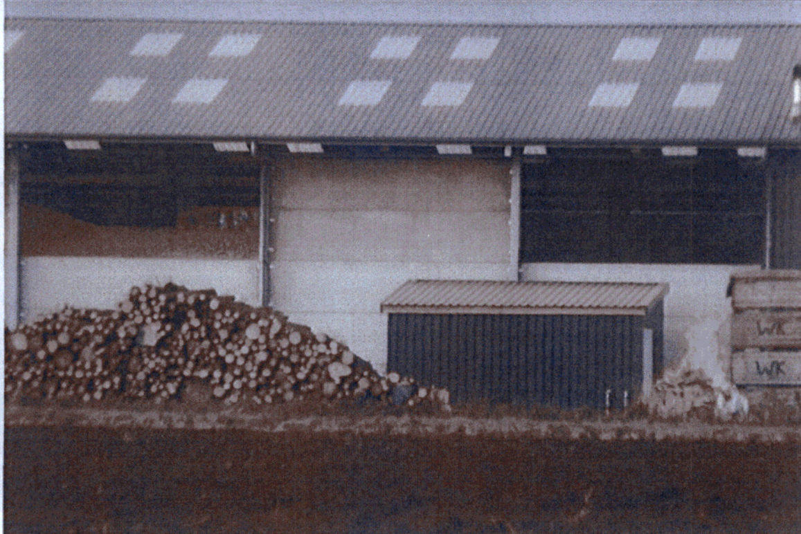
11. Piperdam Biomass Facility. Fire safety hazards (Note positioning of site generator and fuel tank in upper image & unattended bonfire in lower image)
