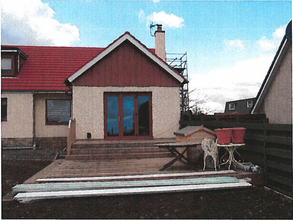
WORKS AS VIEWED FROM THE EAST
