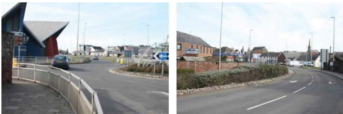
Photographs 7 & 8 – Footpath adjacent to A92 Burnside Drive/ East Mary Street Roundabout with visi-rail and deterrent measures to prevent crossing movements past the central reserve and nearside carriageway
