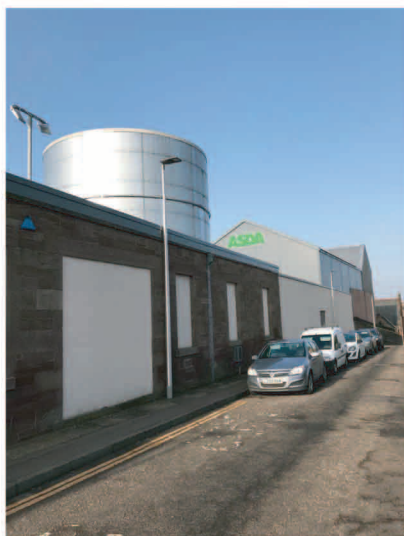
showing a large metal cylinder not appropriate architecture in a conservation area
