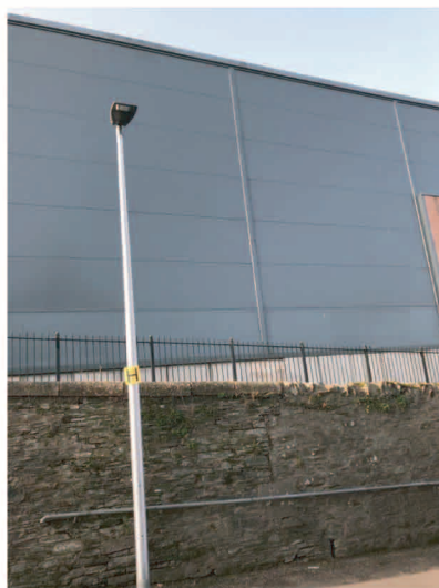
mordern sheet cladding panels inconsistant with a conservation building materials
