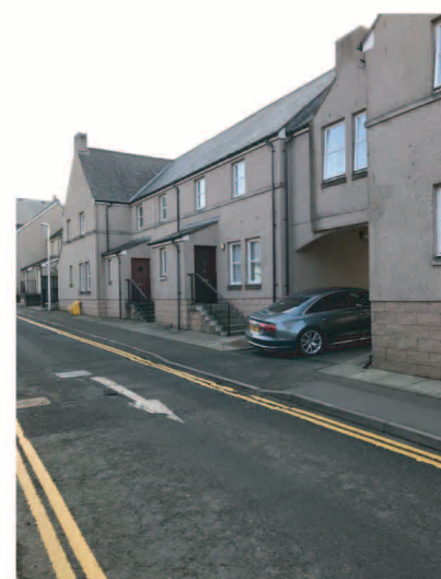
Pink harled apartments which are out of place when compared to the tradioal brown stone buildings
