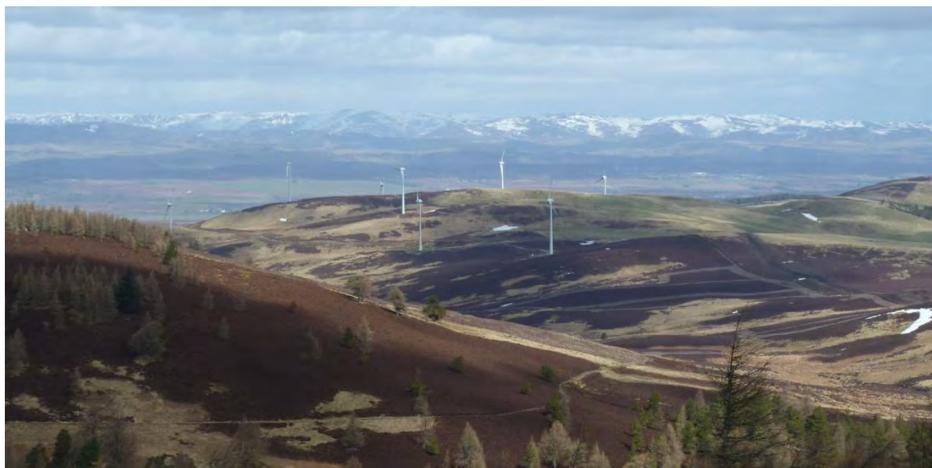
Ark Hill Windfarm
