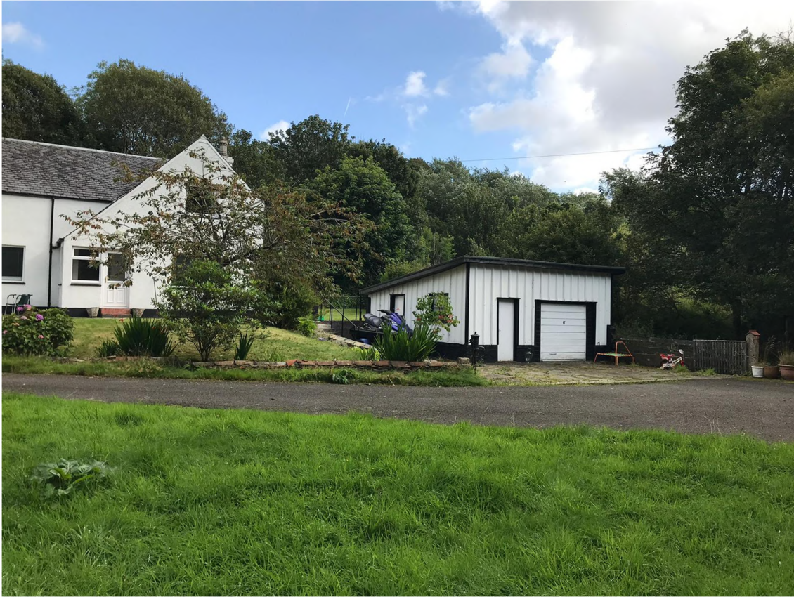
Figure 5: View North of Hawthorn Cottage from Dighty Burn
