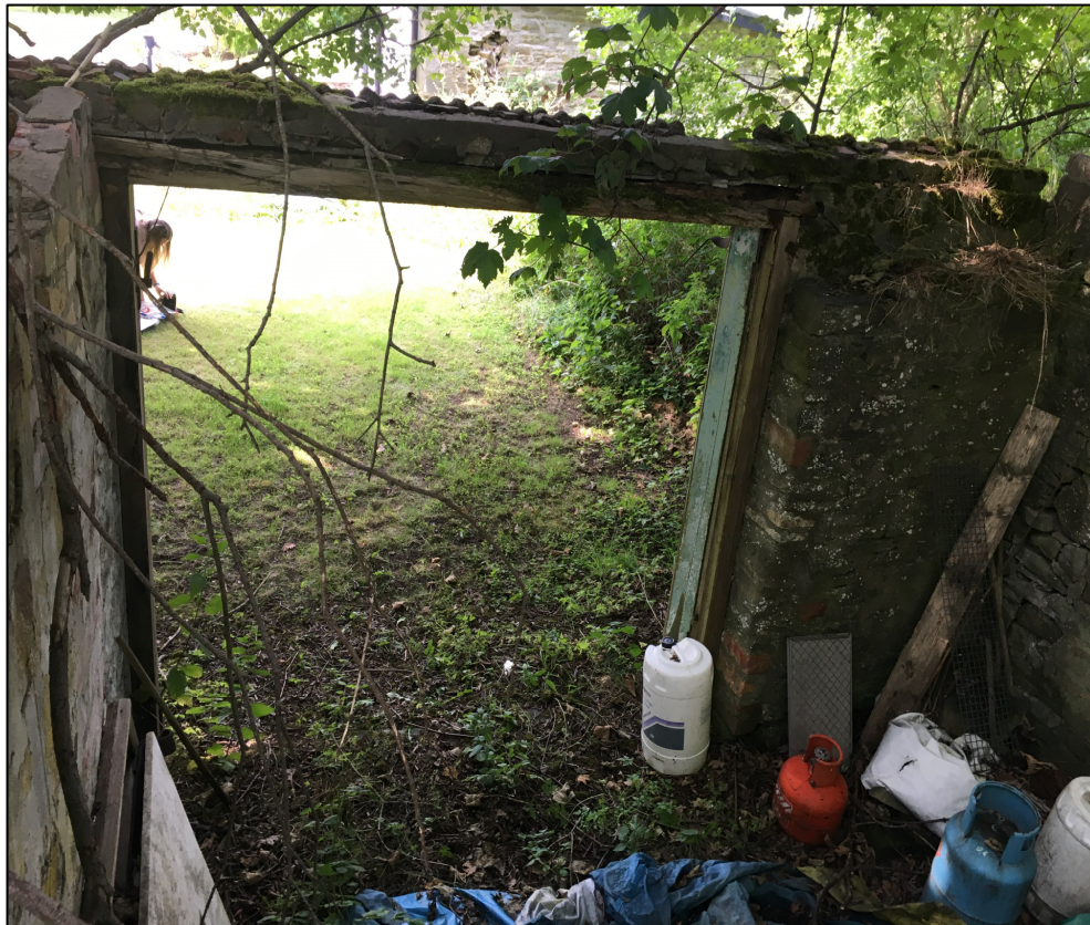
Figure 3. Shell of building.
