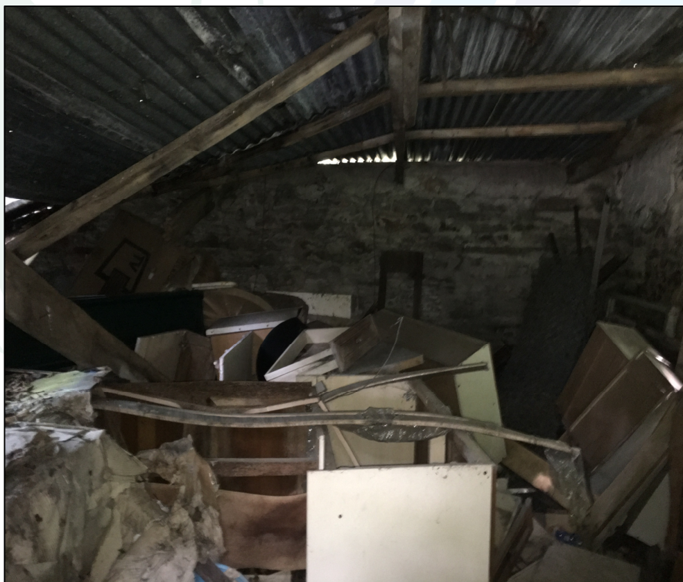
Figure 4. Corrugated sheeting onto wooden joists
