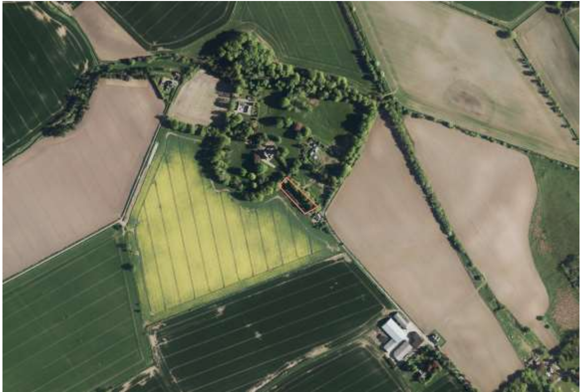
1.5 Figure 3: Site Ownership illustrates the applicant's land ownership edged blue, within the context of the planning application site, edged red.
